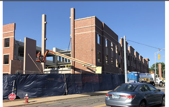
Willard & DiLoreto Garage construction
