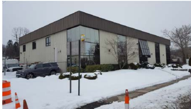
View of the subject property's office/warehouse as seen from Old Newtown Road. This photo was taken facing east. The trees within the Drainage Right of Way area had already been removed prior to this photo being taken.
