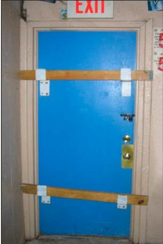
The image shows a blue door with a red "EXIT" sign above it. Two wooden bars are placed horizontally across the door, one near the top and one near the bottom, which would prevent the door from being opened.
