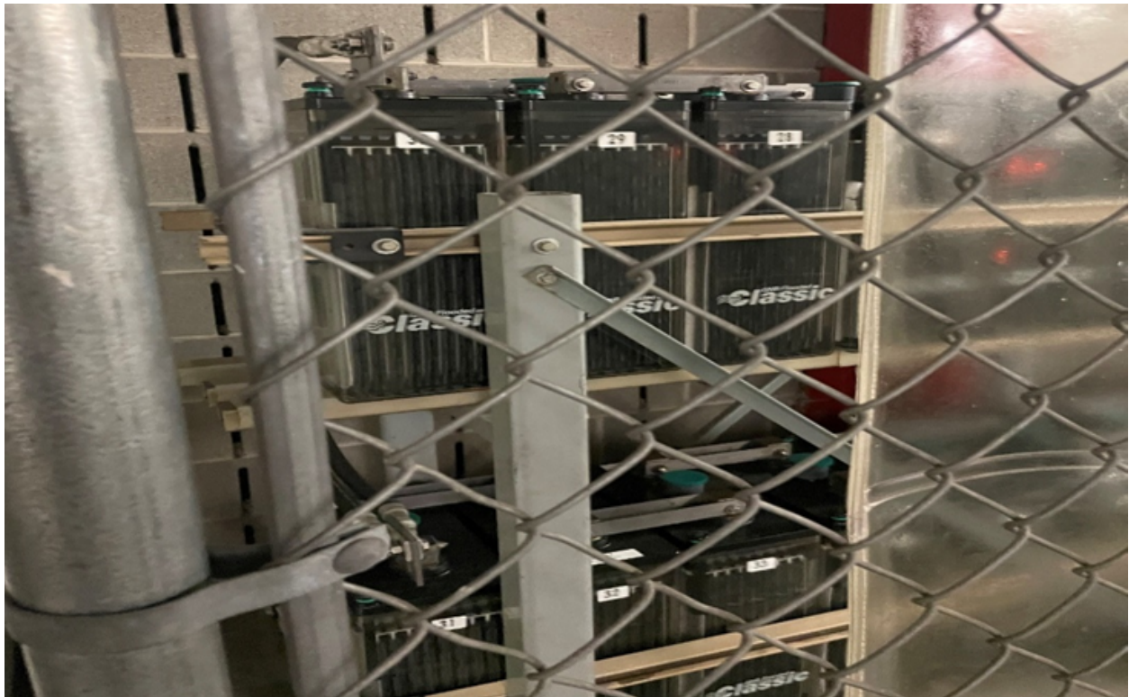
Figure 8: 125VDC Lead Calcium Batteries
