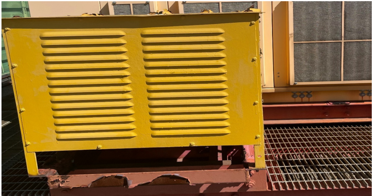
Figure 3: Neutral Grounding Resistor NGR
