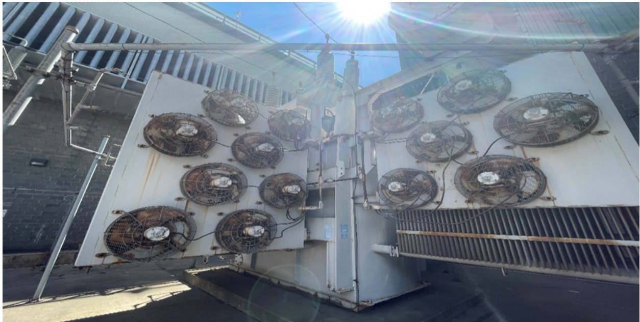
Figure 1: 115kV main utility transformer
