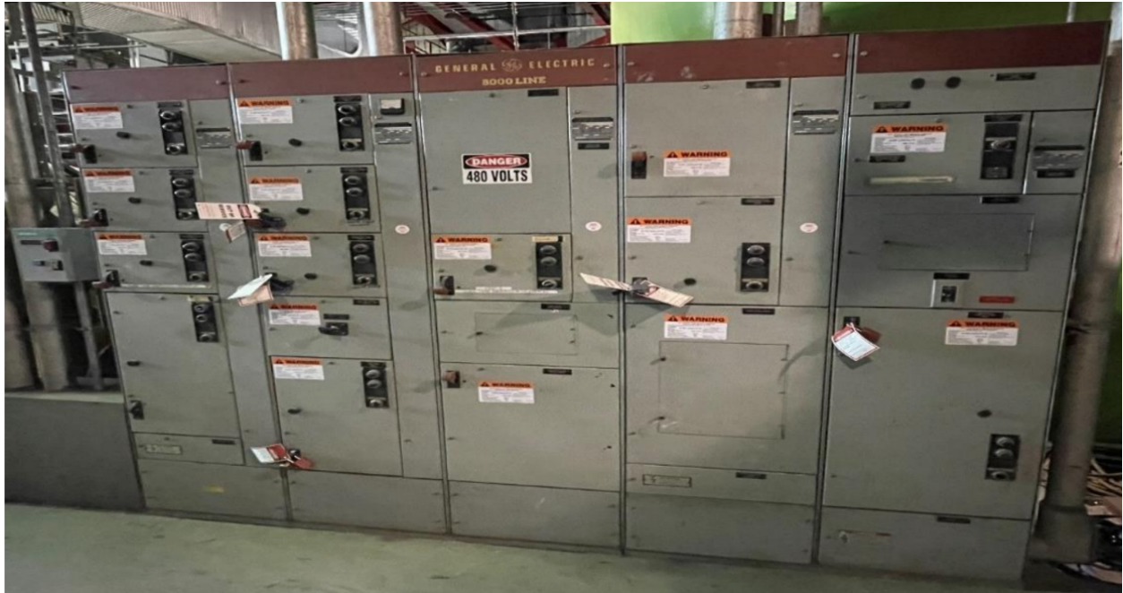
Figure 15: Gas turbine motor control center MCC-GT
