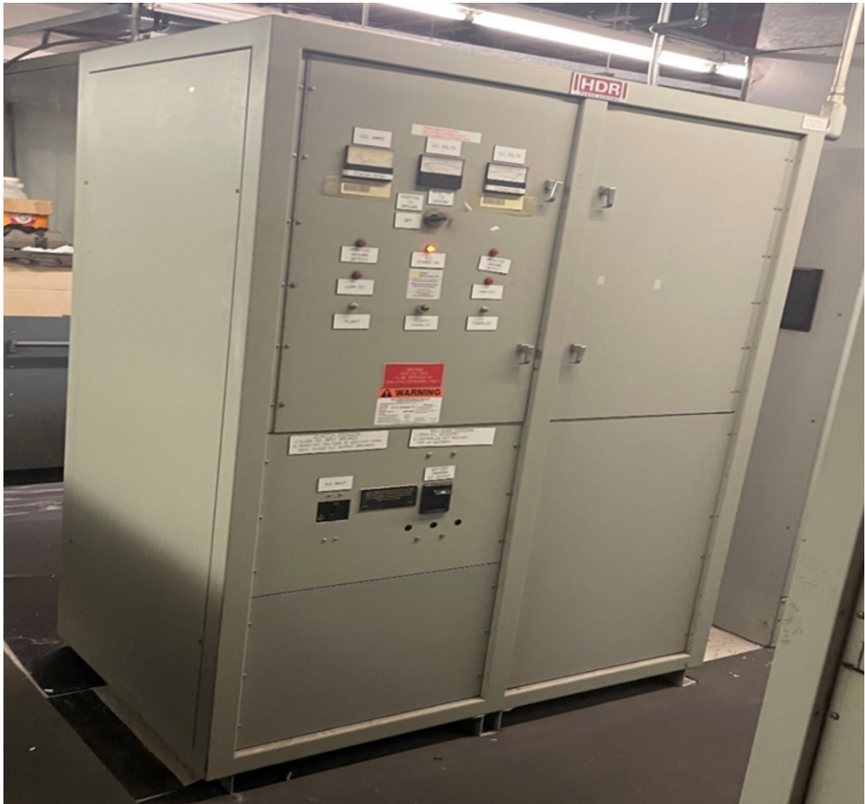
Figure 7: 125VDC Battery charger and Inverter
