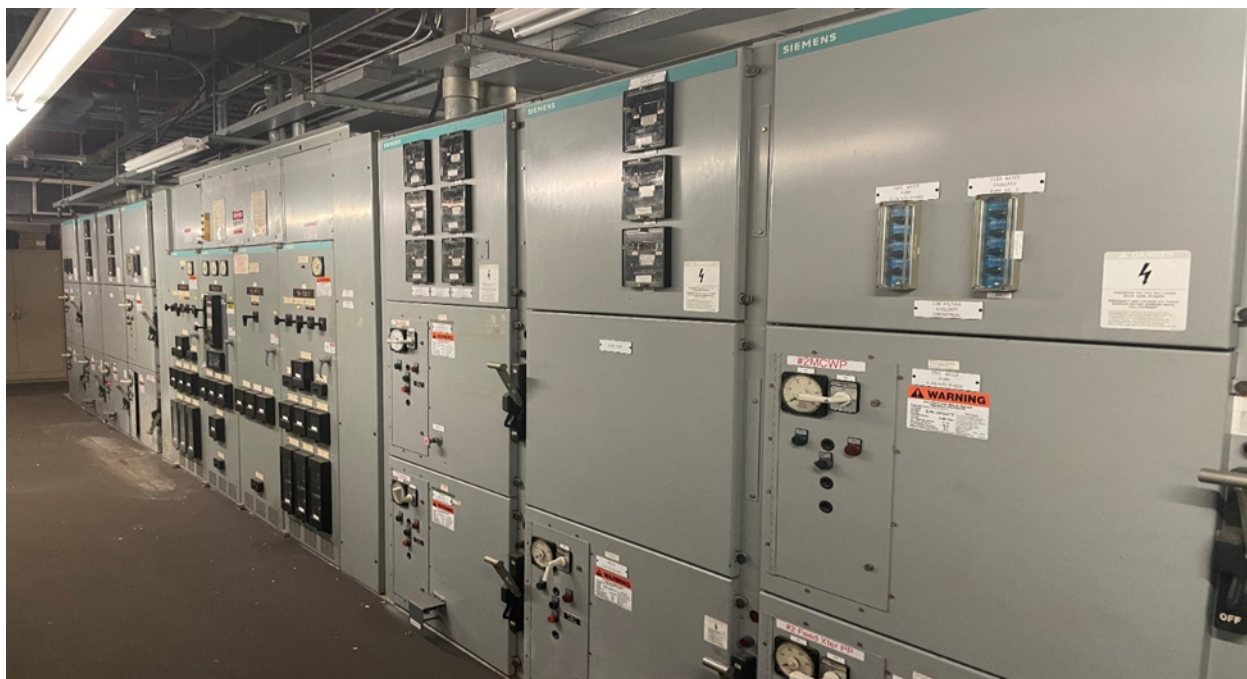
Figure 10: Existing electromechanical relays
