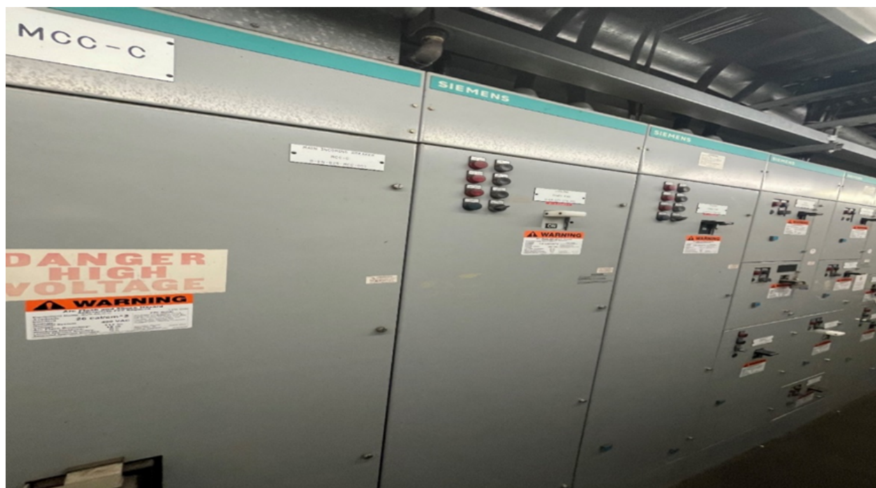
Figure 13: 480V motor control center MCC-C
