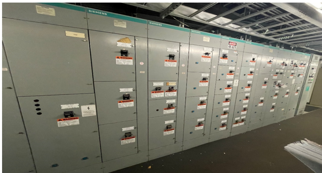
Figure 14: Motor control center MCC-D
