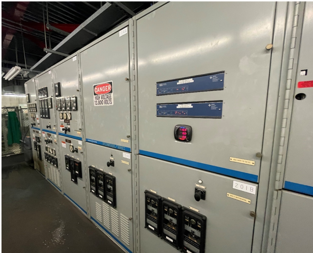
Figure 6: 13.8kV Main Switchgear
