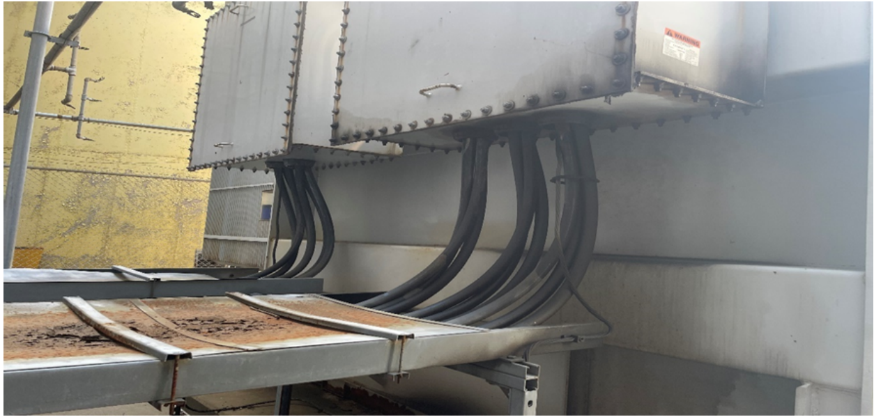
Figure 2: 13.2kV cables on Transformer 51L-1X secondary
