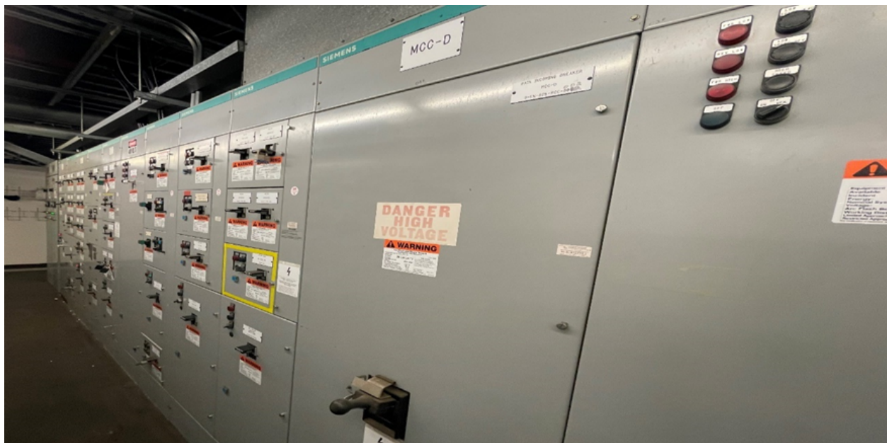
Figure 12: motor control center MCC-D
