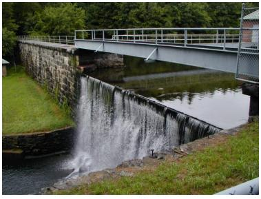
While the Dam will be raised 4' the spillway and normal reservoir level will remain unaltered
