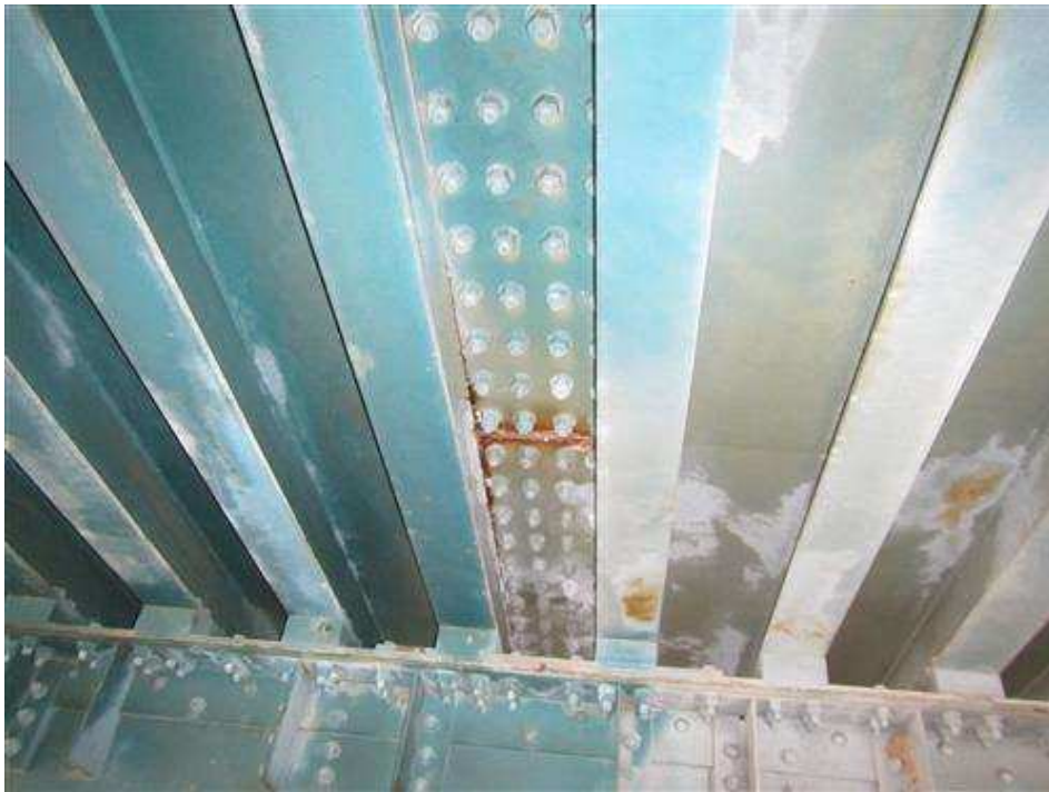
Panel 4, bay 11, deck splices near floorbeam 5, note the laminated rust at the ends of the splice plates.
