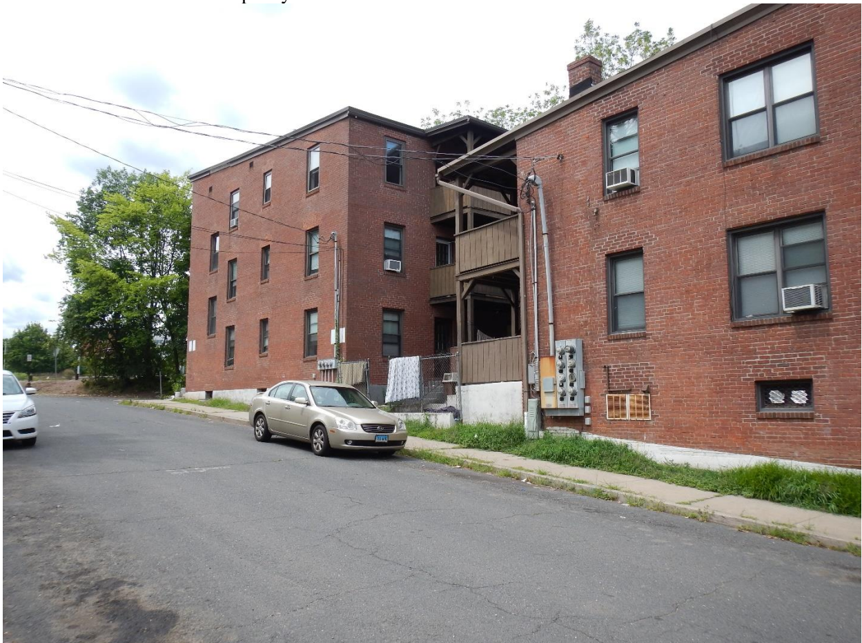
Photo 2: Image of 61 East Main Street with front building to right, potentially affected rear apartment at center, and Route 17 on-ramp at far left.
