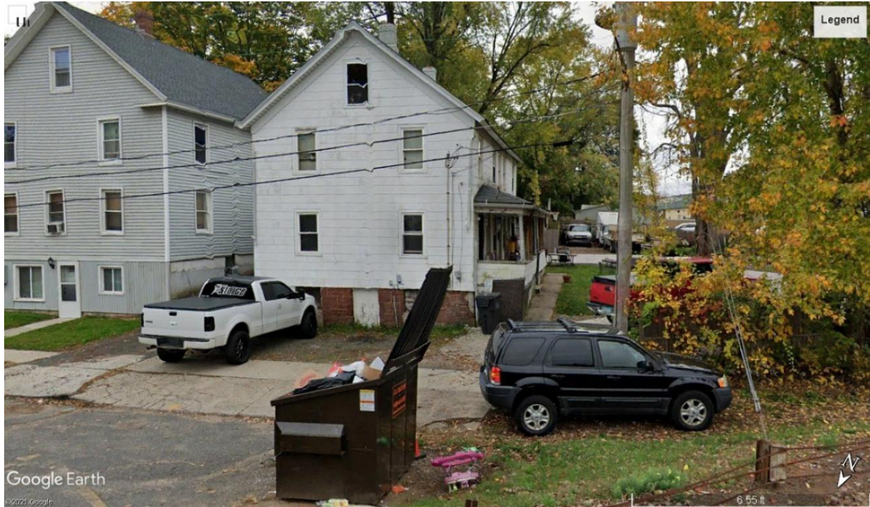
Photo 3: 7 Flower Street (at center) view from Route 17 ramp.
