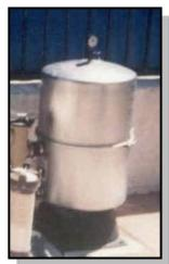
should be disassembled and the filter grids removed, cleaned and inspected for damage. This should be done every 2 to 3 months depending on pool bather load. The local sewer district may also require D.E. separators for these filters, especially if the pool exceeds 2000 square feet. Safer filter media such as Perlite may also be used in D.E. filters. Check with the manufacturer's standards.
