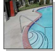
**GUTTERS** are found at large municipal and club pools or older pools built before 1960. Gutters serve two functions: trap debris and scum from the surface of the water and provide a handhold for bathers.
