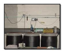
return line downstream, or after the filter and heater, in order to reduce any possible chemical damage to the equipment.
