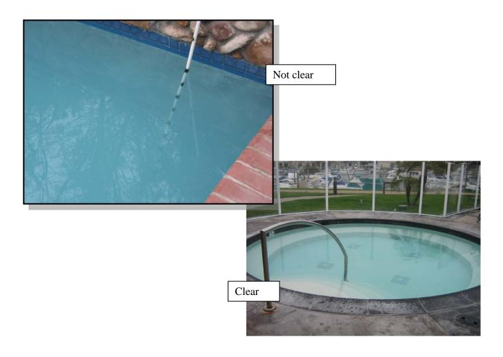
**SAFETY TIP!** Check daily to see if you can easily see the main drain covers from the deck. If the drain is not visible, close the pool until the water clarity improves.
