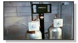
primarily used only to feed carbon dioxide to lower pH. If you use gas feeders, be sure that the gas tanks are securely fastened to the wall to prevent them from falling over when accidentally bumped or during an earthquake.
