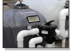
for routine maintenance is lower water quality and water clarity because a sand filter can only trap particles larger than 25 microns for high-rate and 50 microns for rapid-rate. Zeolite has been demonstrated as a material that may be used as a replacement for traditional silica sand. This material has been shown to filter down to 3 to 5 microns. Check with the manufacturer for existing sand filters.
