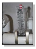
and maintenance of the flow meter is important to ensure accurate readings. San Diego County has "hard water" which over time can cause a calcium layer to form inside the flow meter, causing the flow meter to get stuck. Check the flow meter routinely.
