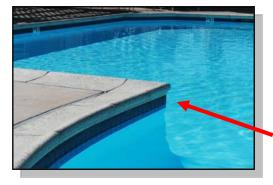
**COPING** around the pool is usually a series of bull-nosed stones that slope away from the pool. This helps keep the pool clean by directing water on the deck away from the pool. Coping also functions as a handhold for bathers and must hang over the pool wall at least 1 inch, but not more than 2 inches. It is not to exceed 2 ½ inches in thickness.
