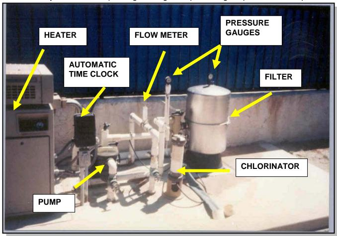
This section provides a brief and general description of the components of a recirculation, filtration and disinfection system of a 30,000 to 40,000 gallon swimming pool. It discusses the different types of filters and disinfection systems that are commonly used in San Diego County.
