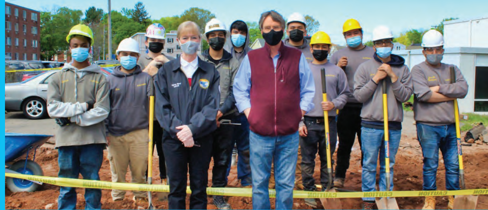
Eli Whitney Technical High School electrical students helped to install West Haven's first charging kiosk for electric cars.
