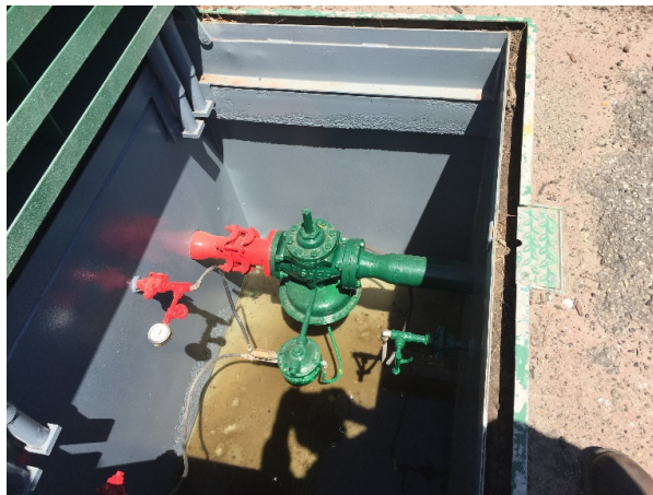
Exhibit 25 - Color-coding for Regulator stations
