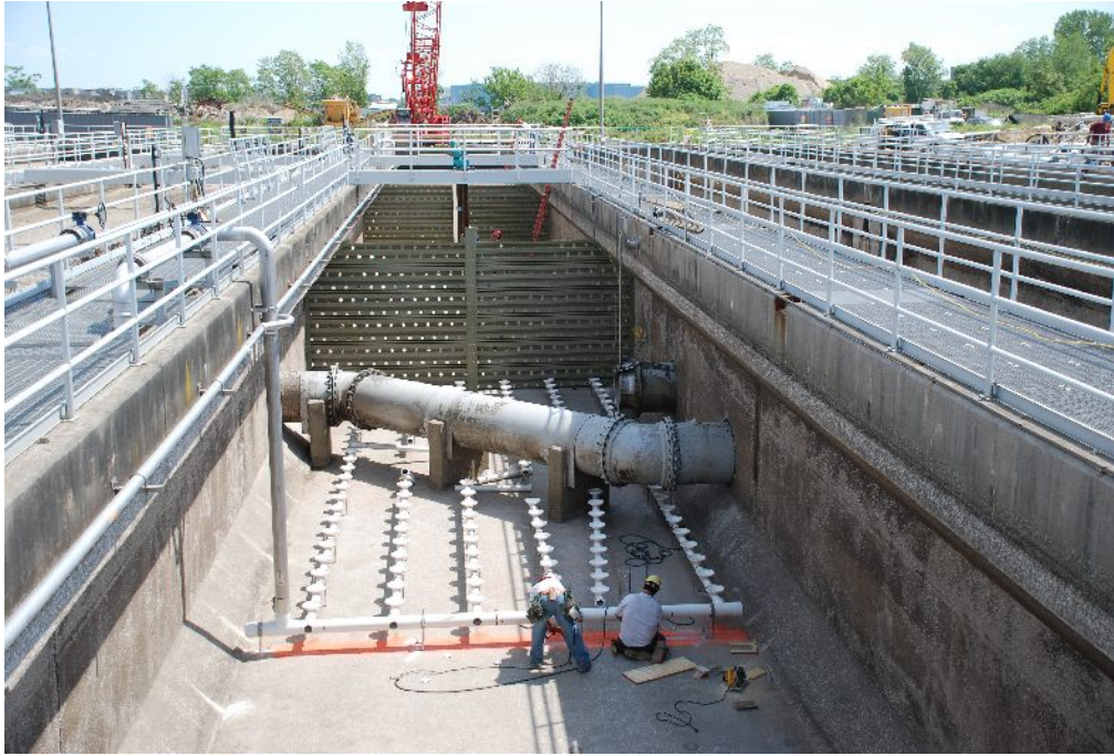
Stratford Wastewater Treatment Facility Aeration Tank Diffuser Installation
