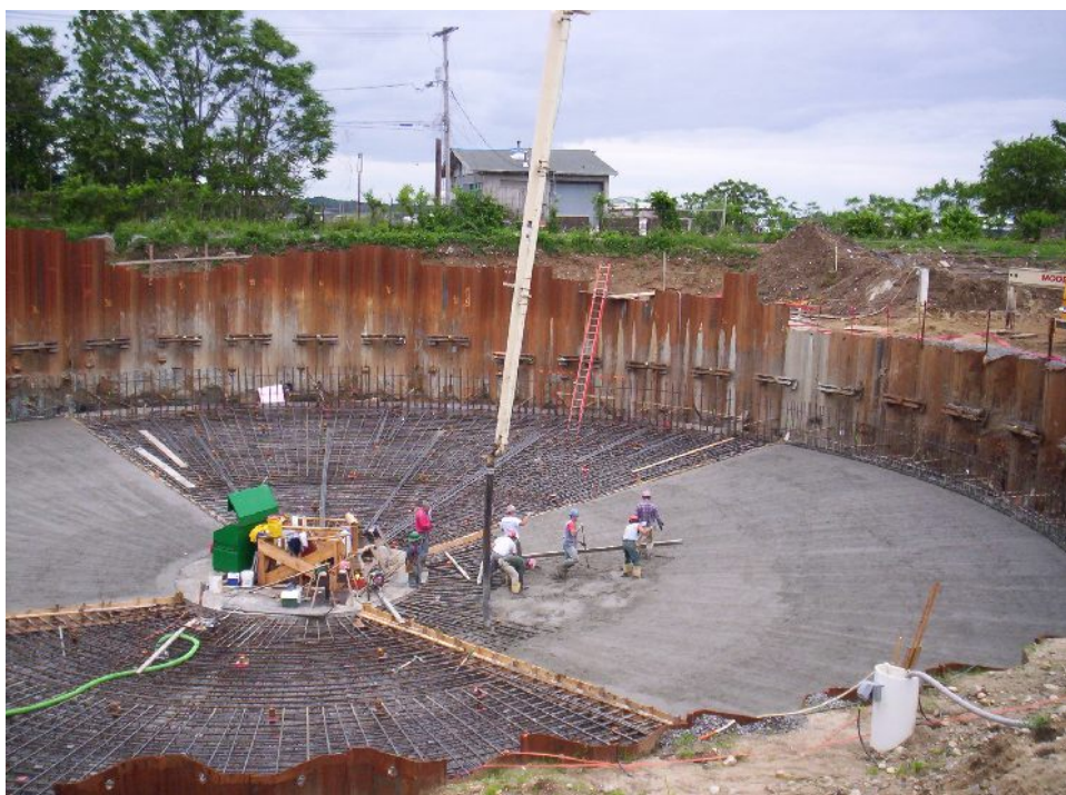
Stratford Wastewater Treatment Facility Clarifier Slab Placement
