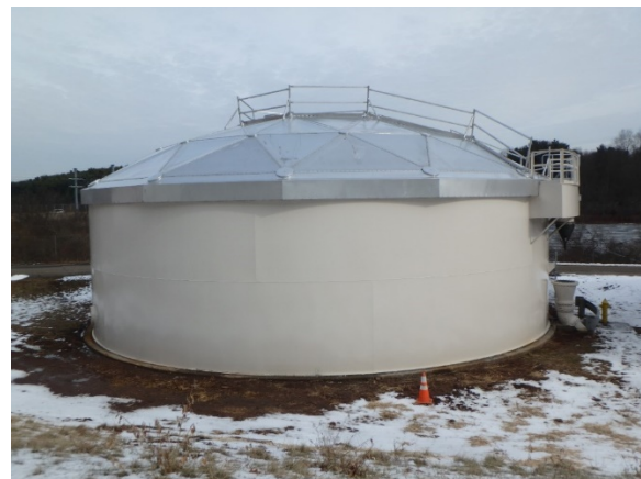
RWA – Lake Saltonstall Tank Improvements – Tank #2
