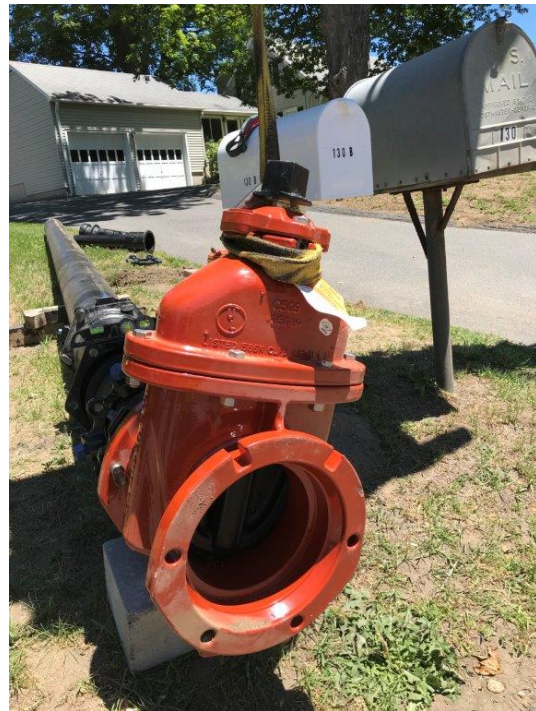
Bethel – Water Main Installation
