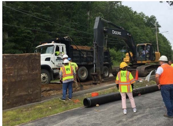
Norwich Public Utilities- Sprague Emergency Interconnection Pipe Trench Excavation Work
