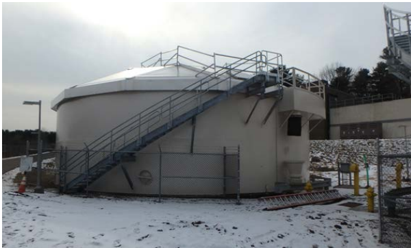
RWA – Lake Saltonstall Tank Improvements – Tank #1
