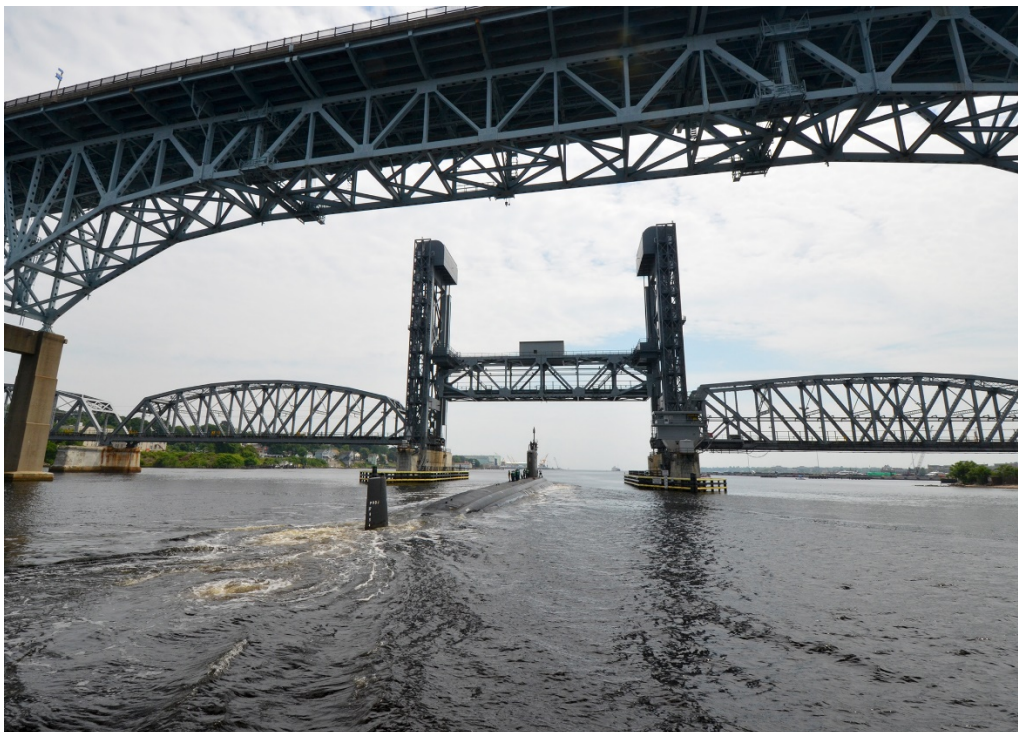
Gold Star Bridge, Thames River
