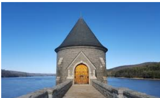
Barkhamsted Saville Dam
