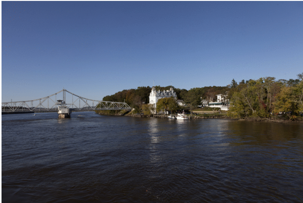
East Haddam Swing Bridge on the Connecticut River
