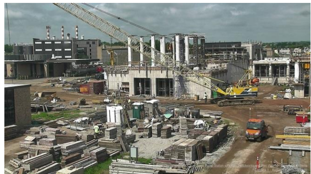
Metropolitan District Pump Station Construction
