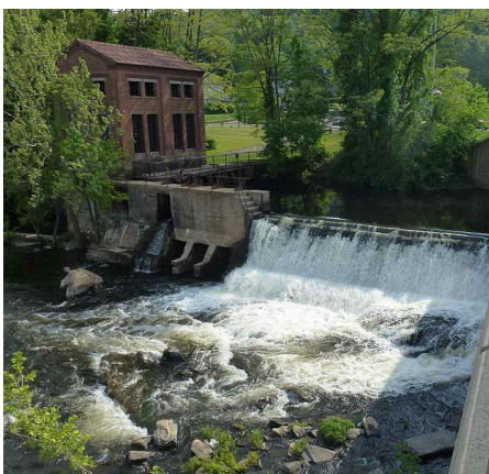
Farmington River Spillway in Collinsville
