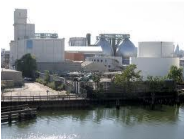
GNHWPCA East Shore Sewage Treatment Plant
