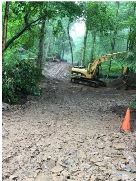
Guilford Mulberry Point – Site Work-Water Main
