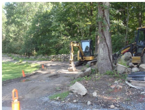
Bethel – Water Main Installation
