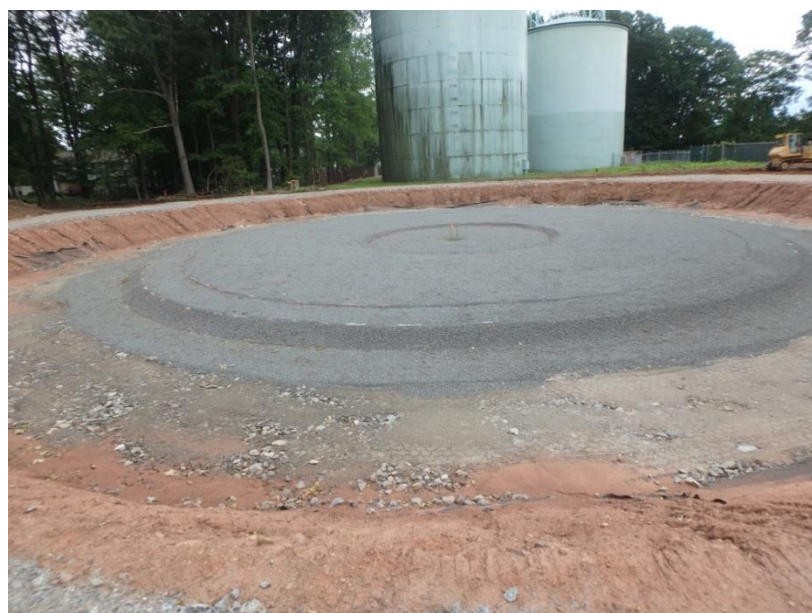
Southington Mill St. – Tank –Foundation Excavation
