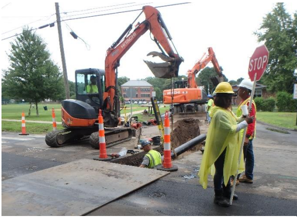
MDC – Garden St. water main installation
