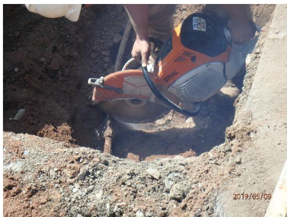
MDC – Removal & replacement of water service line, Bond Street project
