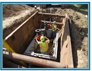
Bolton Lakes: Installation of low pressure sanitary sewers as part of the small community project to protect the Bolton Lakes.
