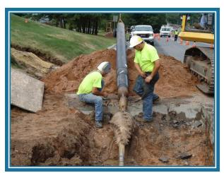
Bolton Lakes: Directional drilling to install pipe with minimal disturbance to surface features (such as State Route 44)
