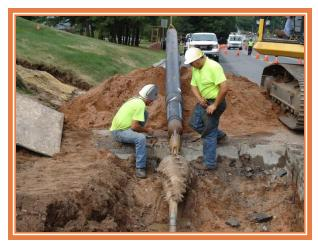
Bolton Lakes: Directional drilling to install pipe with minimal disturbance to surface features (such as State Route 44) (Photo courtesy of Fuss & O'Neill, Inc.)
