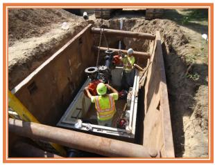
Bolton Lakes: Installation of low pressure sanitary sewers as part of the small community project to protect the Bolton Lakes. (Photo courtesy of Fuss & O'Neill, Inc.)
