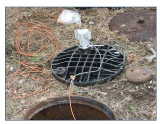
MDC RF III – New Remote Reading Radio Frequency Device Attached to Underside of Meter Pit Cover
