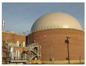
Norwich WPCF: Energy recovery project, utilizing waste gases from the treatment plant to generate electrical power (Photo courtesy of Norwich DPU)
