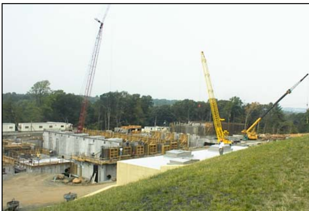
New Britain Plant Construction Site New Britain, CT
