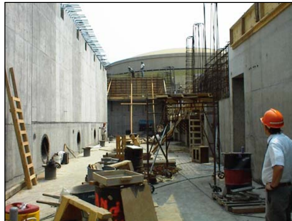
New Britain Plant Construction Site New Britain, CT
