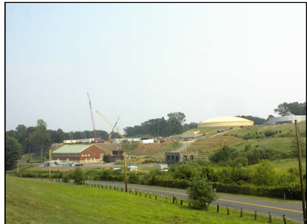
New Britain Water Facility, New Britain, CT
