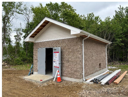
SECWA SEVEN OAKS PROJECT, PUMP STATION, MONTVILLE
