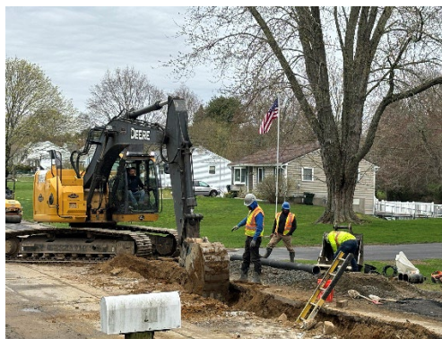
NPU CARIBOU PROJECT, WATER MAIN TRENCH, NORWICH
