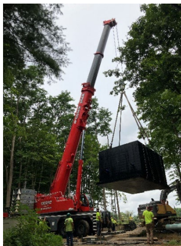
AQUARION CRAIGMOOR PFAS PROJECT, VAULT SETTING, RIDGEFIELD
