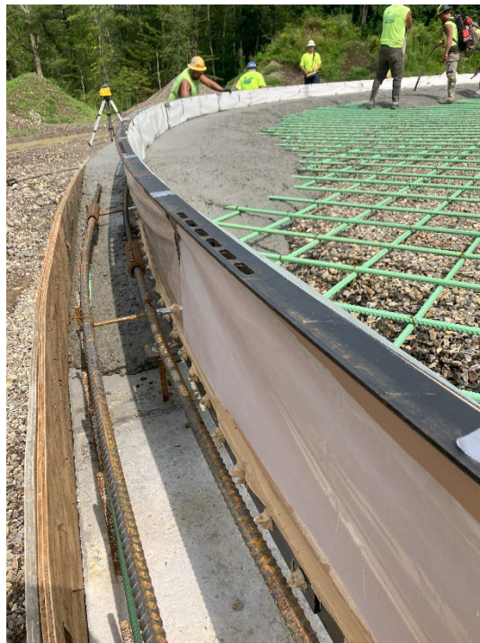
WALLENS HILL STORAGE TANK, WINCHESTER
