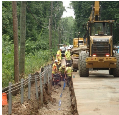
CONNECTICUT WATER COMPANY, TRENCH, MADISON
