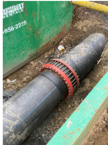
WATERBURY WATER DEPARTMENT, THIRD WATER TRANSMISSION MAIN SLIPLINING, FUSING MACHINE (LEFT PHOTO), MECHANICAL RESTRAINT (CENTER PHOTO), HIGH DENSITY POLYETHYLENE PIPE (RIGHT PHOTO), WATERBURY
