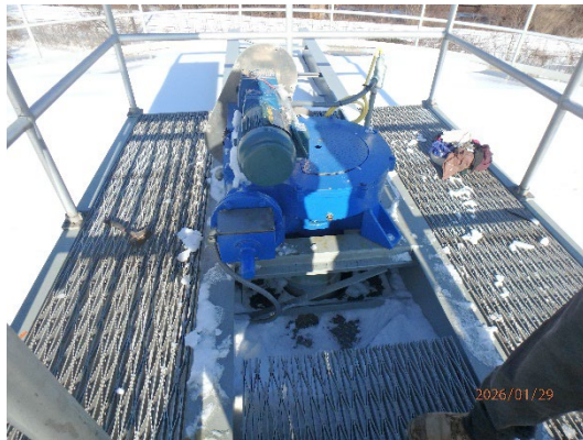
REGIONAL WATER AUTHORITY, LAKE SALTONSTALL NEW GRAVITY THICKENER DRIVE (LEFT PHOTO) NEW SLUDGE PUMPS (RIGHT PHOTO), EAST HAVEN
