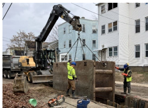
METROPOLITAN DISTRICT COMMISSION, WATER MAIN TRENCH , HARTFORD
