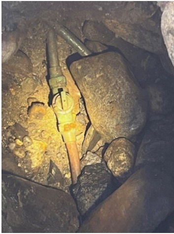
NORWICH PUBLIC UTILITIES, SERVICE LINE AT CURB STOP (LEFT PHOTO) POTHOLING TO VERIFY MATERIAL SERVICE LINE (RIGHT PHOTO), NORWICH
