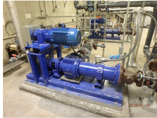
REGIONAL WATER AUTHORITY, LAKE SALTONSTALL NEW GRAVITY THICKENER DRIVE (LEFT PHOTO) NEW SLUDGE PUMPS (RIGHT PHOTO), EAST HAVEN
