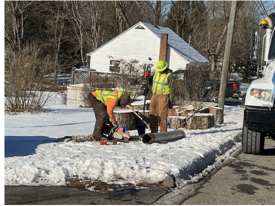
NORWICH PUBLIC UTILITIES, SERVICE LINE AT CURB STOP (LEFT PHOTO) POTHOLING TO VERIFY MATERIAL SERVICE LINE (RIGHT PHOTO), NORWICH
