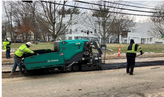
METROPOLITAN DISTRICT COMMISSION, MARSHALL & LAUREL WATER MAIN REPLACEMENT , HARTFORD
