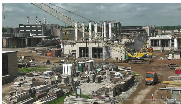
MDC Pump Station Construction
