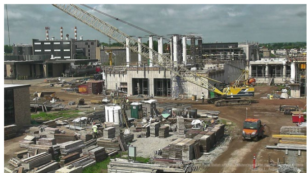
MDC Pump Station Construction
