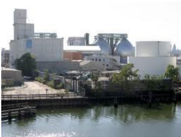
GNHWPCA East Shore Sewage Treatment Plant
