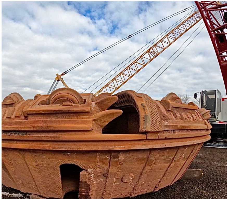
"Iris" the Tunnel Boring Machine for MDC's South Hartford Conveyance & Storage
