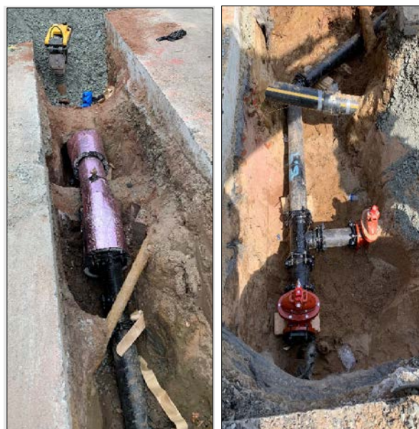
MDC – Buckingham St. Water Main Replacement – Crossing Other Utility Piping
