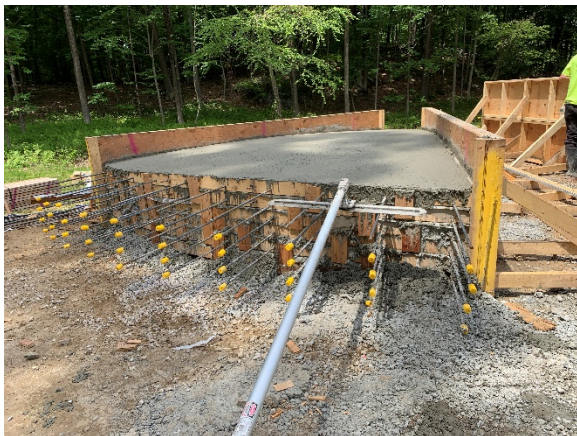
Bethel – Chestnut Ridge Storage Tank Forming of Roof Panels
