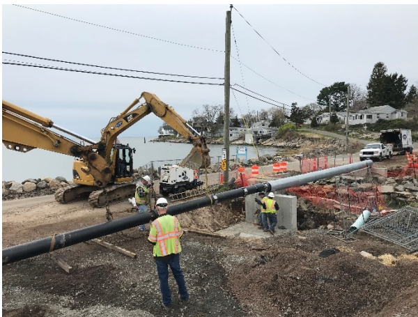
Guilford – Installation of new Water Main crossing over a stream
