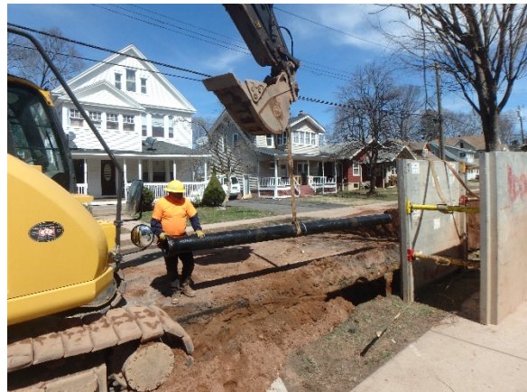
Manchester – Installation of Water Main (above) to Replace Old Stove Pipe Type Water Main (below)
