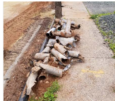
Manchester – Installation of Water Main (above) to Replace Old Stove Pipe Type Water Main (below)
