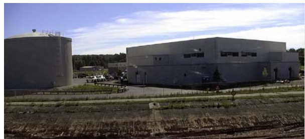
Groton – Newly Upgraded Water Treatment Plant
