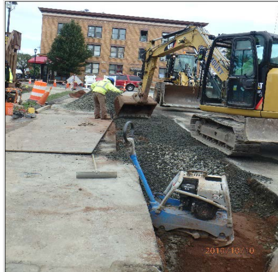
MDC – Replacement of Water Main – Madison Avenue
