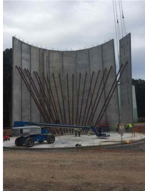
Southington – Mill Street Tank – Installation of side panels
