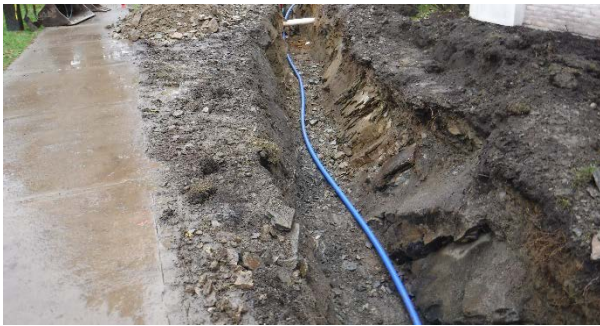
St. Joseph School & Church –Connection to Aquarion Water Company
