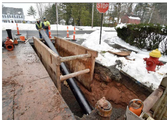
MDC –Webster Hill Water Main Replacement (both photos)
