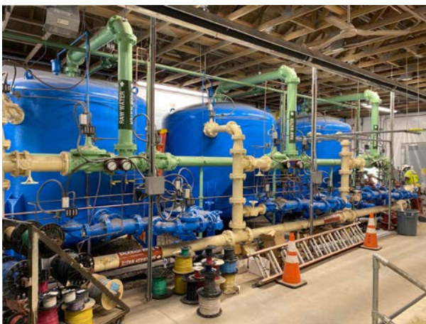
East Lyme – Filtration Treatment Vessels
