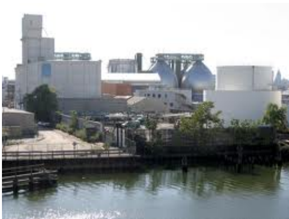
GNHWPCA East Shore Sewage Treatment Plant
