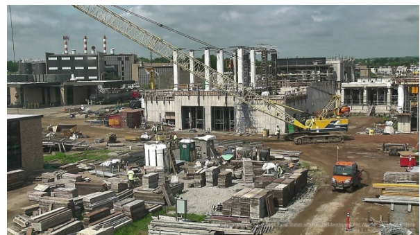
Metropolitan District Pump Station Construction
