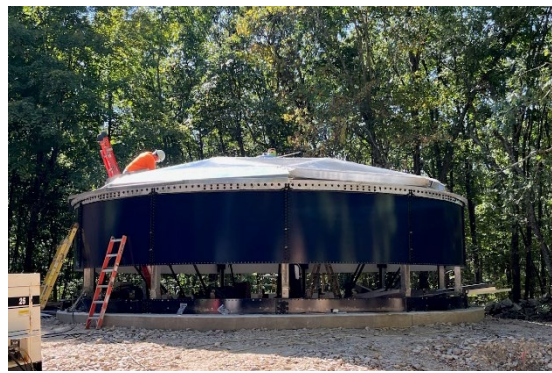
MONTVILLE NEW TANK CONSTRUCTION
