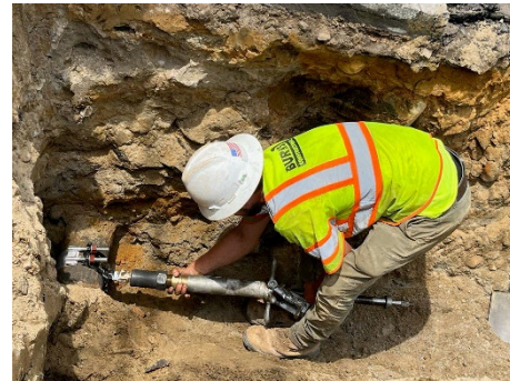
NEW LONDON NEW SERVICE LINE INSTALLATION
