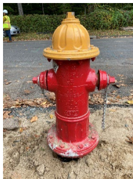
MDC HUBBARD RD WATER MAIN REPLACEMENT - NEW FIRE HYDRANT
