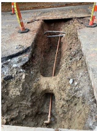
MDC CAPITOL AVENUE PROJECT, NEW SERVICE LINE INSTALLATION
