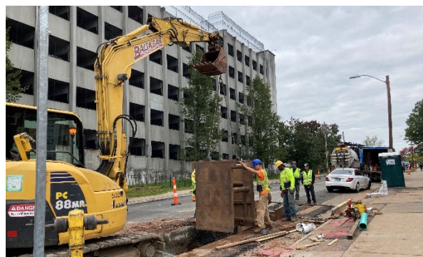
MDC HARTFORD HOSPITAL AREA WATER MAIN REPLACEMENT
