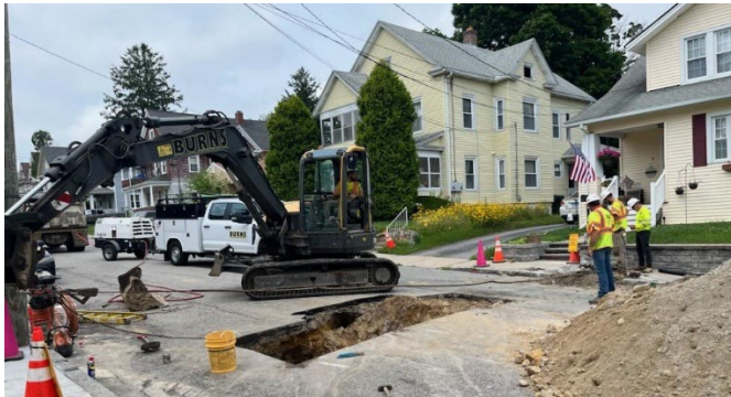
NEW LONDON LEAD SERVICE LINE REMOVAL
