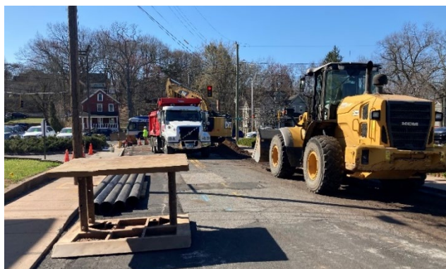
WATER MAIN REPLACEMENT, MANCHESTER CT
