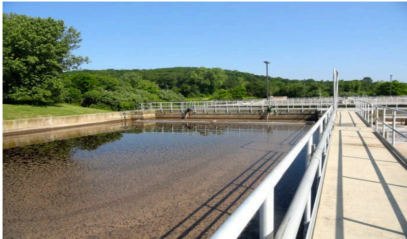
Wastewater Treatment Plant, Montville, CT
