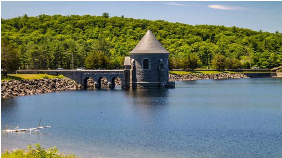
Saville Dam at Barkhamsted Reservoir
