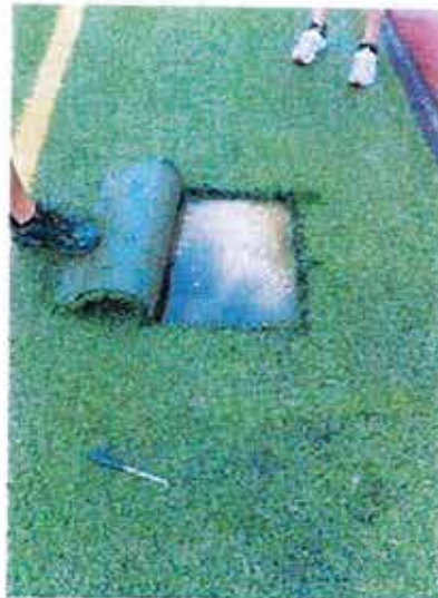
Ponding over stone base
