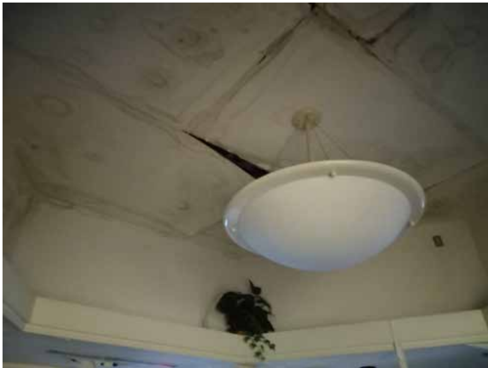
Second floor interior
