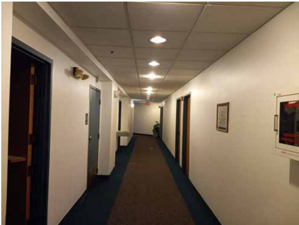
Second floor interior
