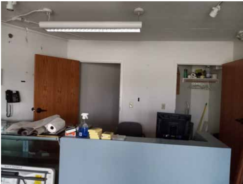
Ground floor interior
