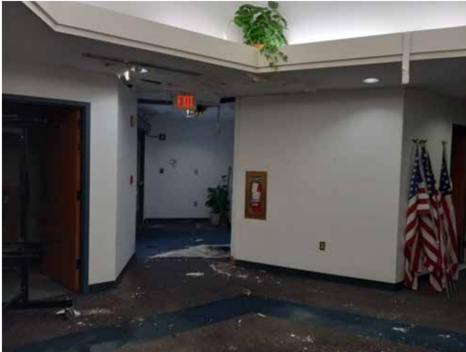
Second floor interior
