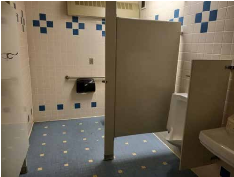
Ground floor interior
