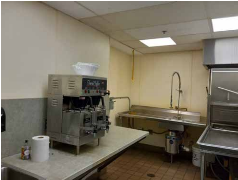
Second floor interior
