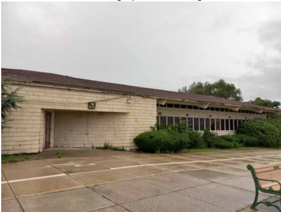
View of existing improvements looking north
