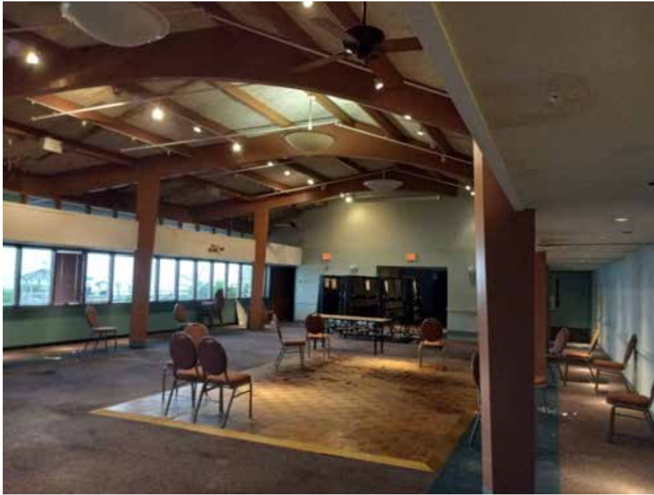
Second floor interior
