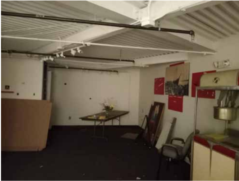
Ground floor interior
