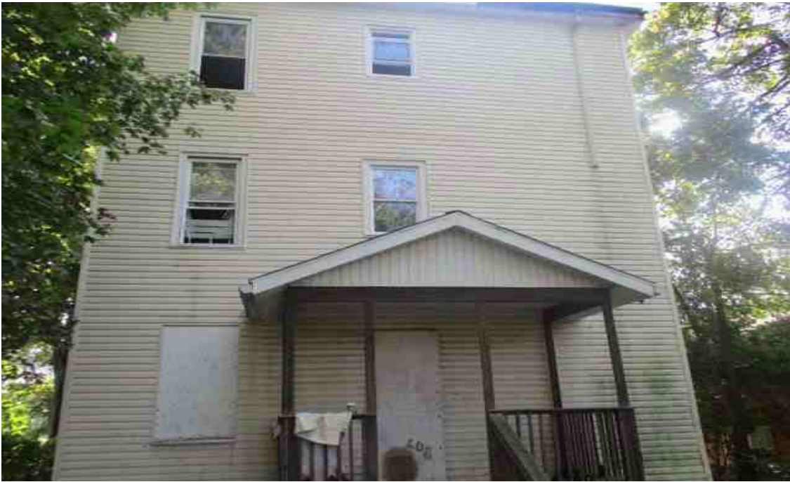
471 Garden Street, Hartford (vacant and blighted)
