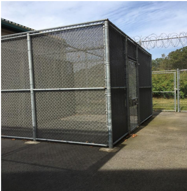
YCI Segregation Unit, Outdoor Rec. Cage and Cell
