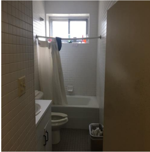
Minor girls' cottage bathroom at YCI
