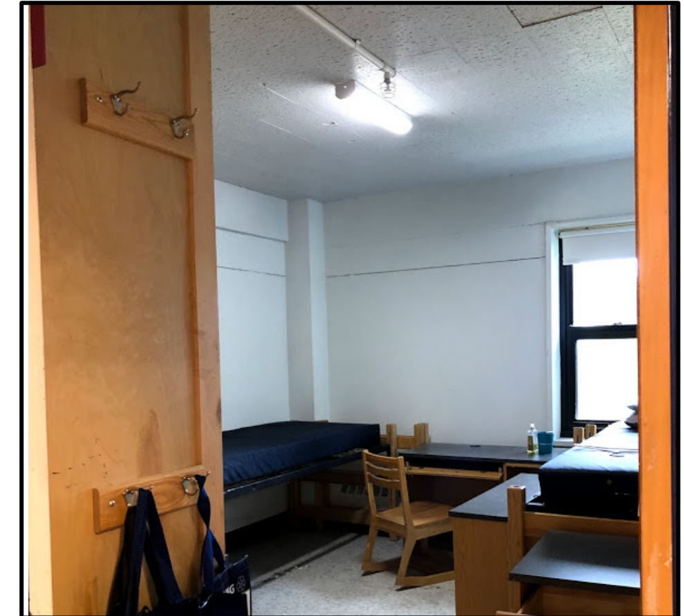
Storrs Residence Hall LED Retrofit
