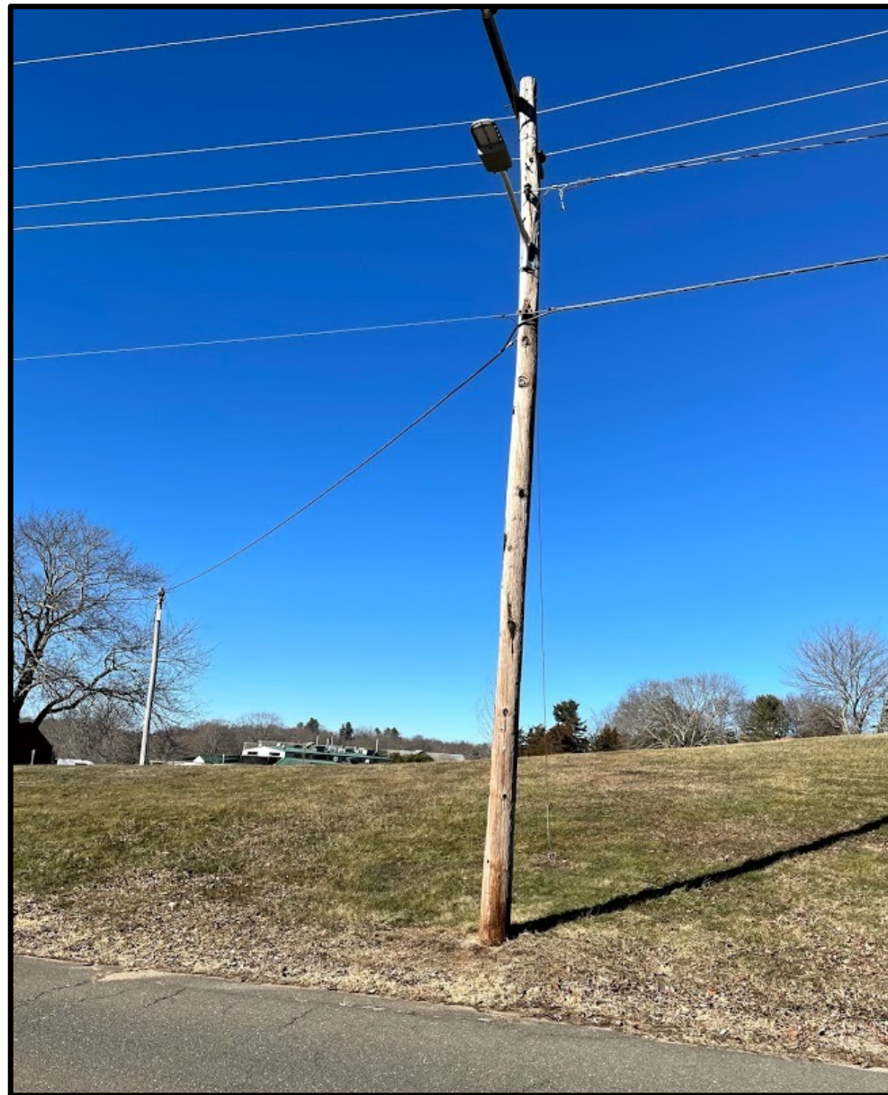
Depot Campus Street Light LED Retrofit
