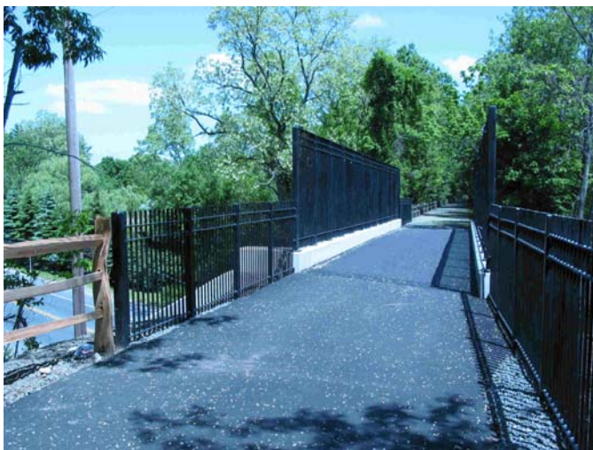
c) Bridge with fencing
