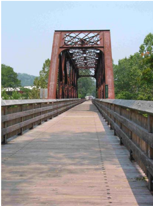
a) Bridge south of Collinsville
