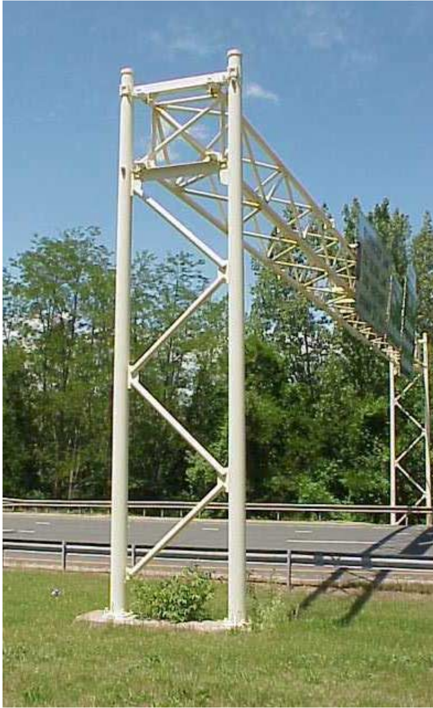
Figure 3 Typical Truss Support
