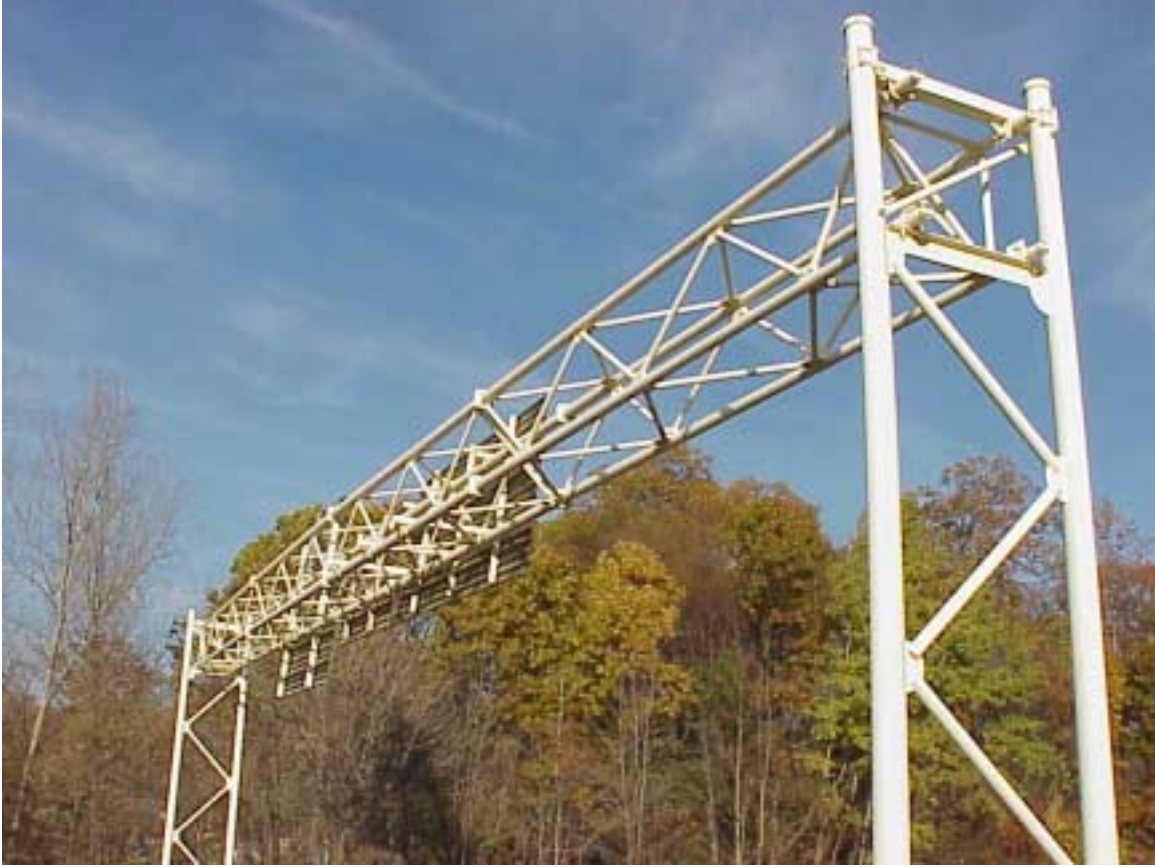
Figure 2 Typical Horizontal Box Truss
