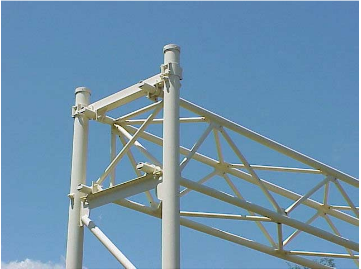
Figure 6 Connection Between Horizontal Box Truss and Vertical Supporting Truss
