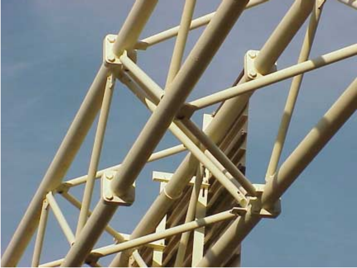
Figure 4 Horizontal Truss Segment Showing Connection Plates
