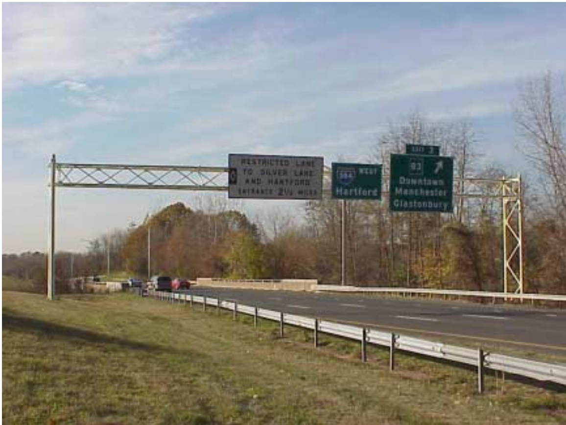
Figure 1 Typical Overhead Truss-Supported Sign Structure
