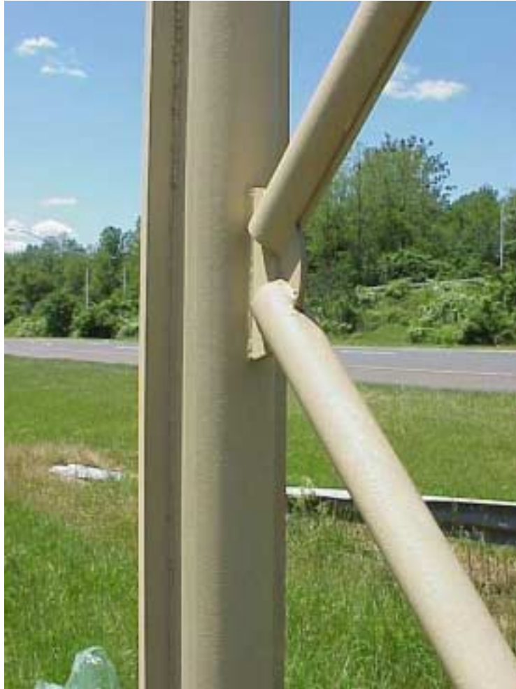
Figure 9 Connection Detail for Reinforced Truss, Showing Stiffener
