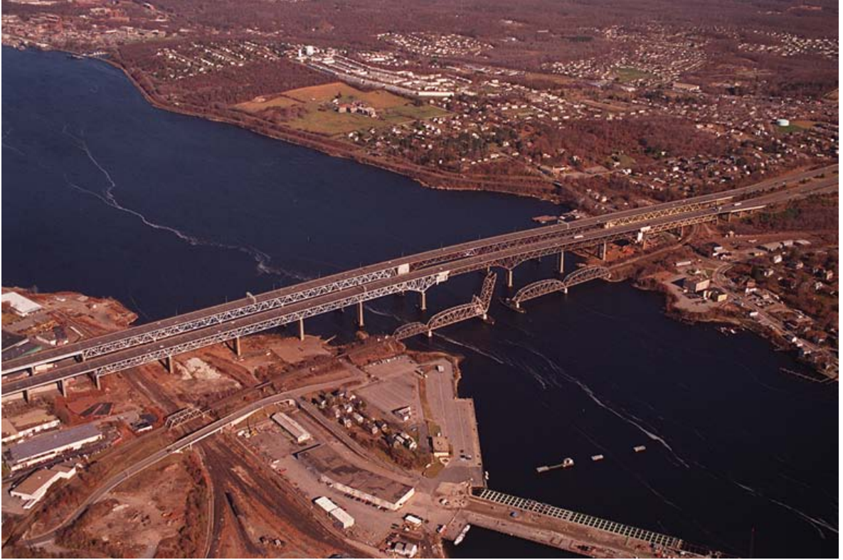
Figure 1. Gold Star Bridge
