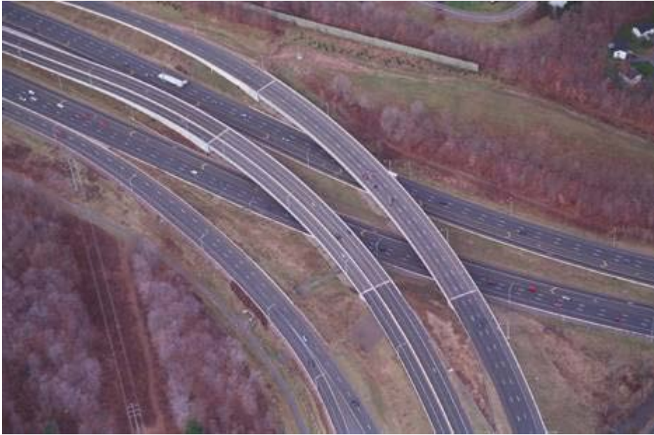
Figure 1. Aerial View of Post-Tensioned Box-Girder Bridge
