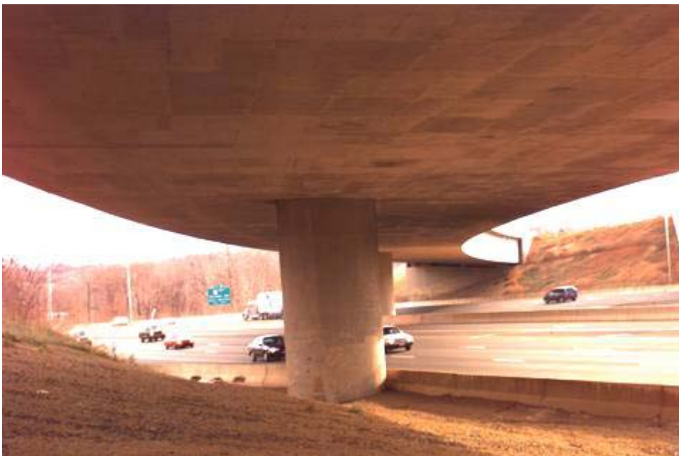
Figure 2. Underside of Post-Tensioned Box-Girder Bridge
