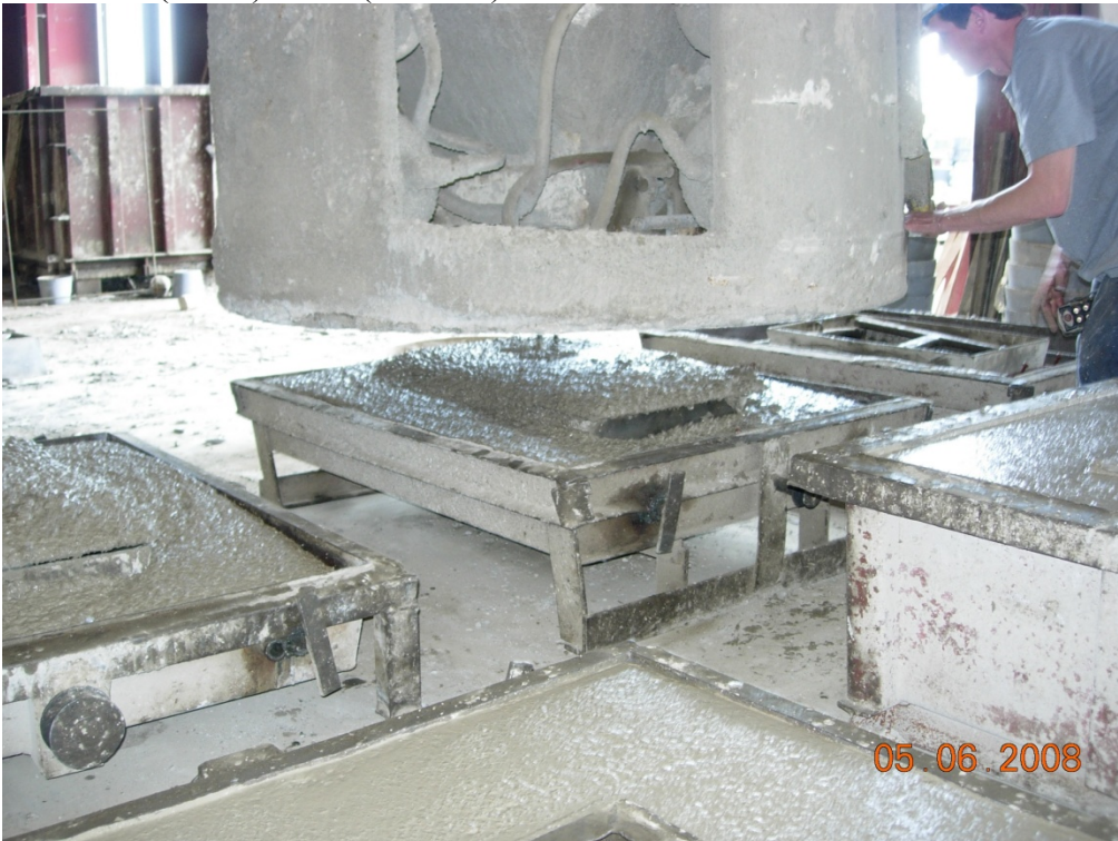
FIGURE 5 - Catch basin top being poured from large bucket.
