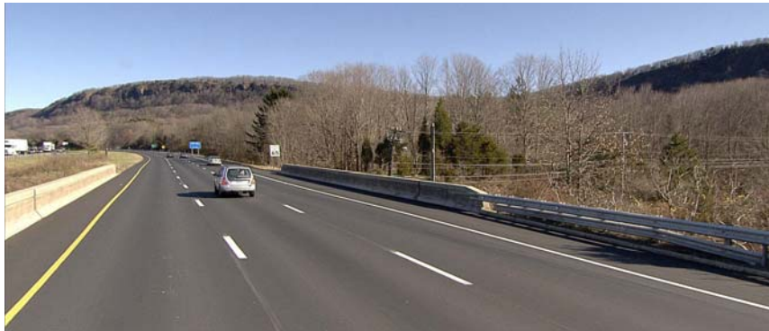
Figure 6: View of the bridge's road surface.
