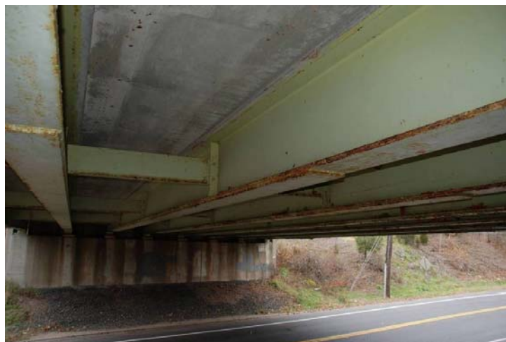
Figure 8: View of the steel girders and underside of the bridge.
