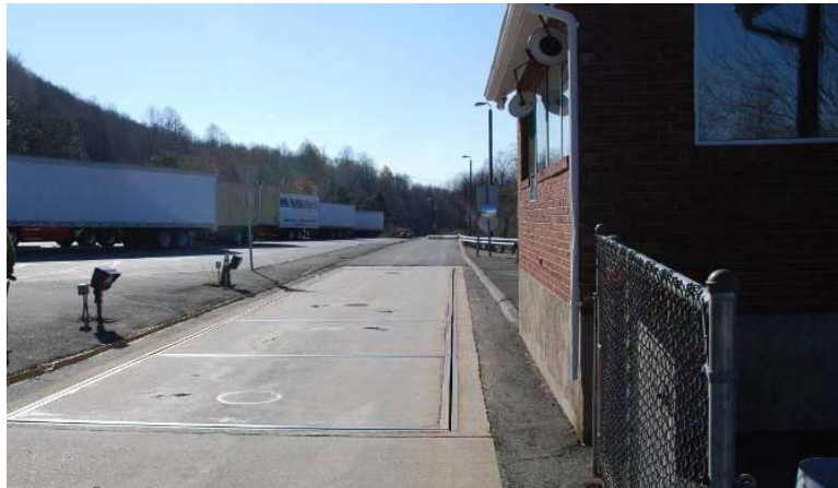
Figure 12: Calibrating the scales at the static weight station.
