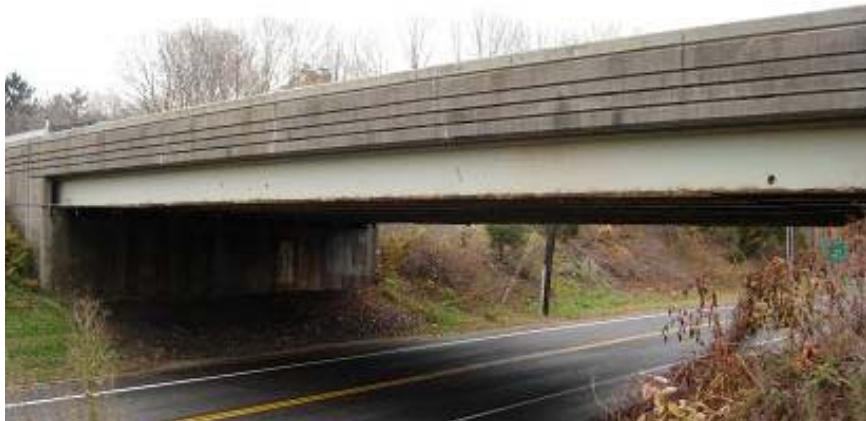
Figure 7: East elevation view of bridge over Baldwin Avenue.
