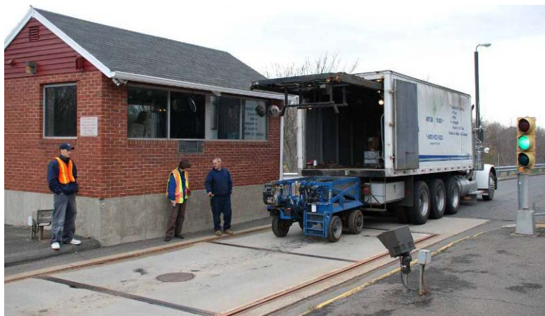
Figure 13: View of the three platforms at the static weigh station.
