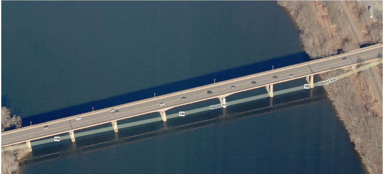
FIGURE 1 Aerial View of Bridge.
