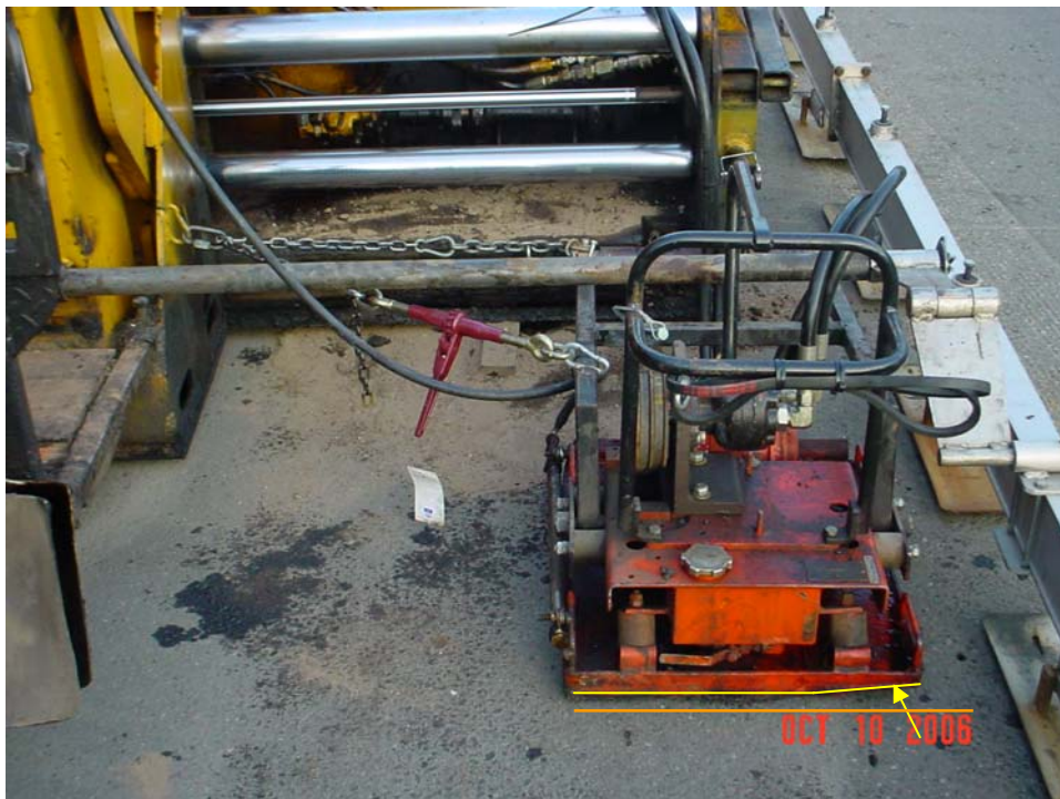
Figure #3 – Wedge Compaction Device and Setup
