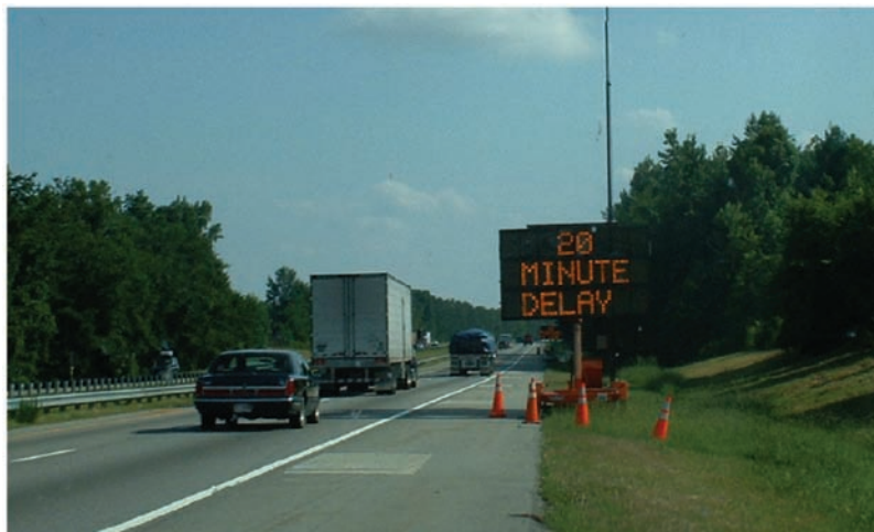
Figure 13: Smart Work Zone Deployment in North Carolina Photo courtesy of International Road Dynamics, Inc.
