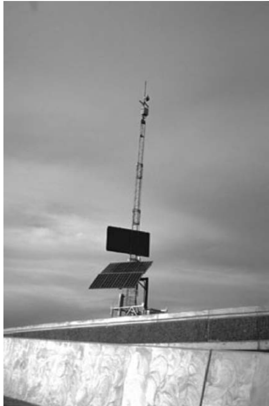
Figure 14 (right): Example of ITS equipment deployed at the Big I Photo courtesy of FHWA (Federal Highway Administration)
