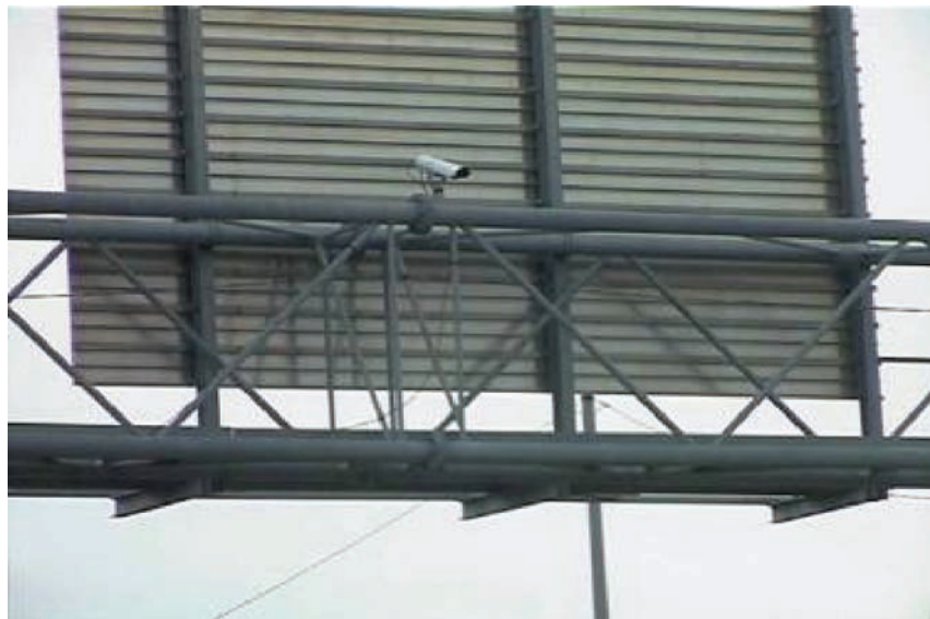
Figure 12: WZSAS Camera Mounted Above Roadway Photo used with permission of Geza Pesti, Texas Transportation Institute
