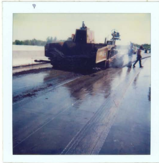
Fig. 3. Placing Class 12 material over waterproofing membrane on bridge deck.
