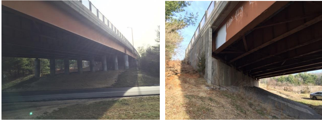
Figure 46: Route 6 Bridge (a) Span and center pier, (b) support at abutment
