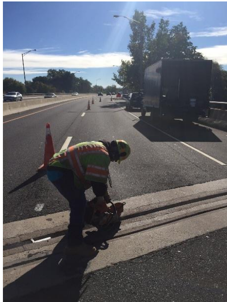
Figure 54: Joint preparation on Route 291 Bridge
