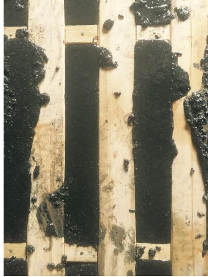
Figure 13: Formwork for polymer modified concrete casting
