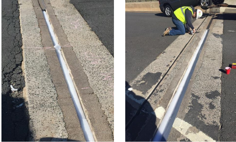
Figure 55: Installation of backer rod and duct tape lining, Route 291 Bridge
