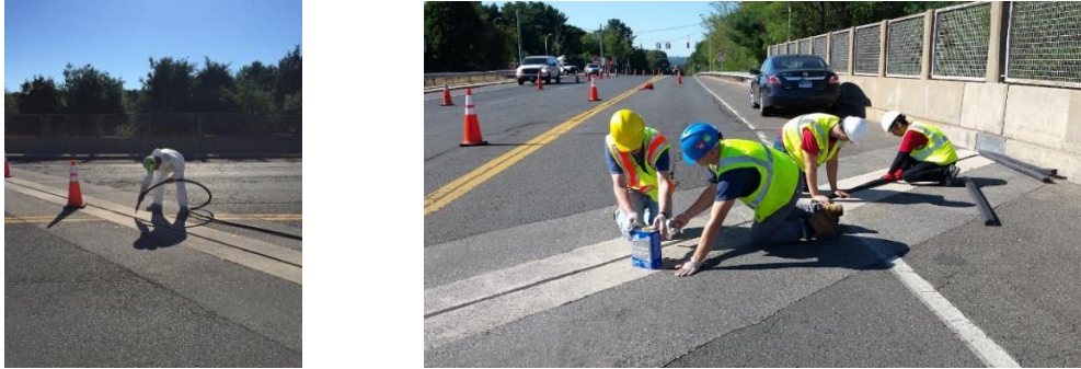
Figure 48: Sand blasting and primer application onto the Route 6 Bridge joint
