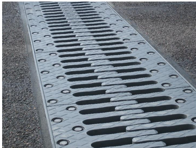
Figure 7: Typical finger joint (Tensa 2015)
