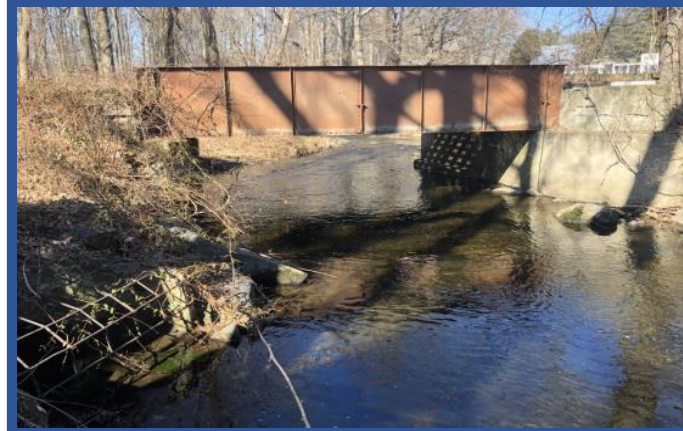
South (Downstream) Elevation
