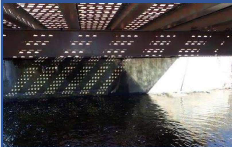
Underside of Superstructure and east abutment.
