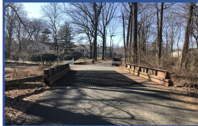
East Approach – looking West over the bridge
