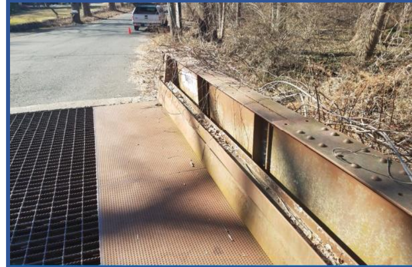
Northern through girder, rub rails, and steel plated sidewalk.
