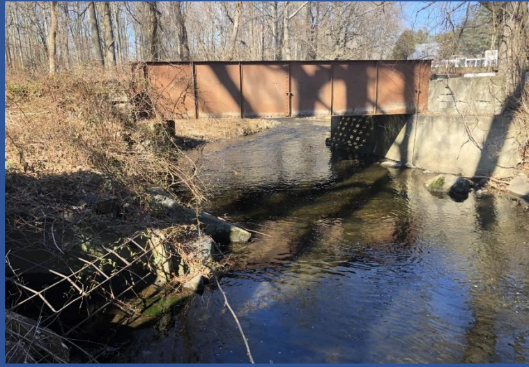
South Elevation (Downstream)
