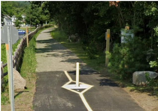
Example Steel Bollard (Moosup Trail in Sterling)
