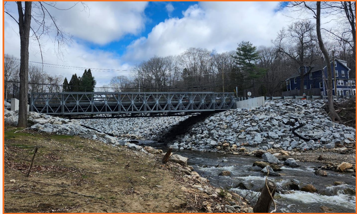
Existing ED Temporary Bridge (ACROW) (From Housatonic River)
