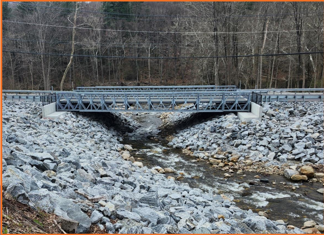
Existing ED Temporary Bridge (ACROW) (From Loughlin Rd)
