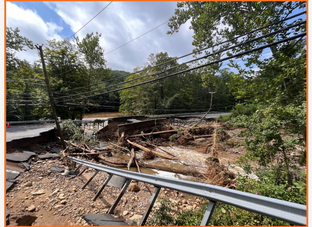
Old Concrete Arch Bridge (after wash-out)
