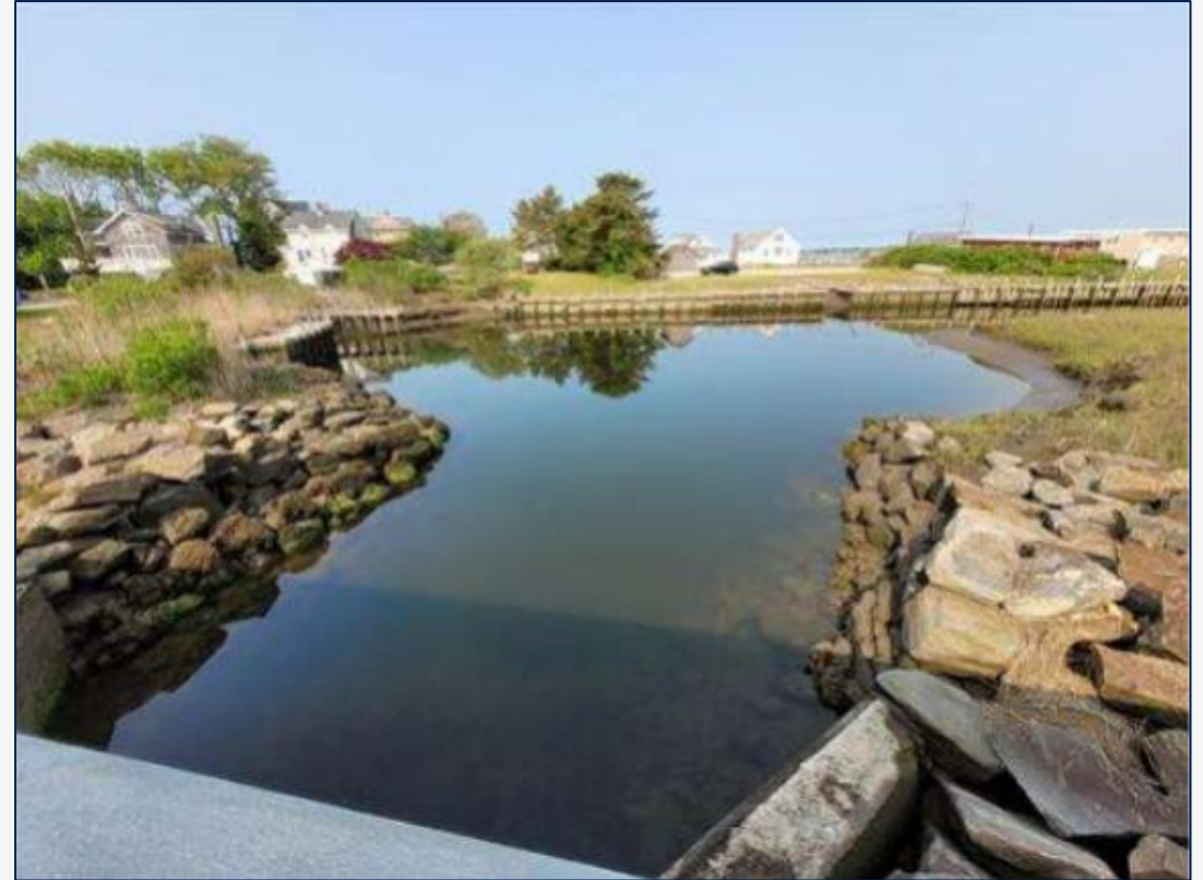
View Downstream of Bridge No. 02708 (Looking West)
