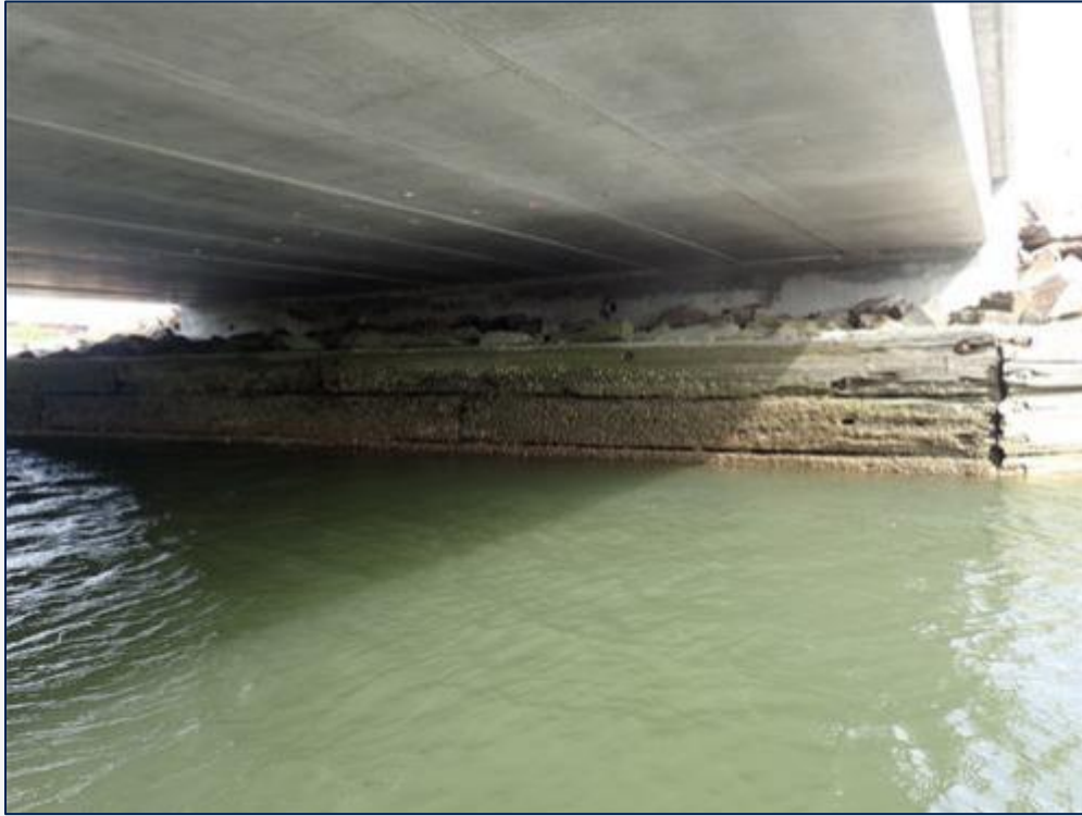
Abutment No. 1 (Looking North)
