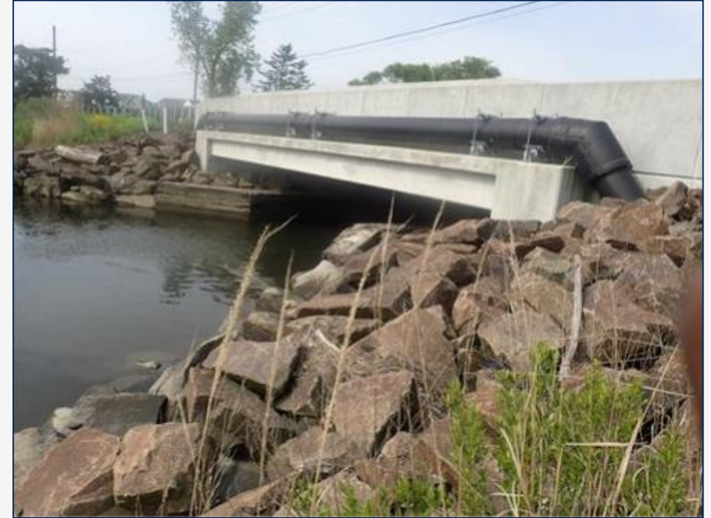
Elevation View (Looking West)
