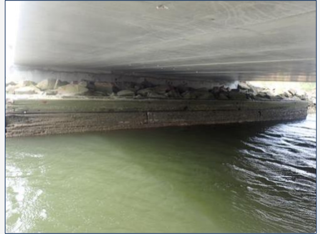
Abutment No. 2 (Looking South)
