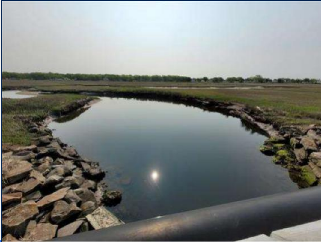
View Upstream of Bridge No. 02708 (Looking East)
