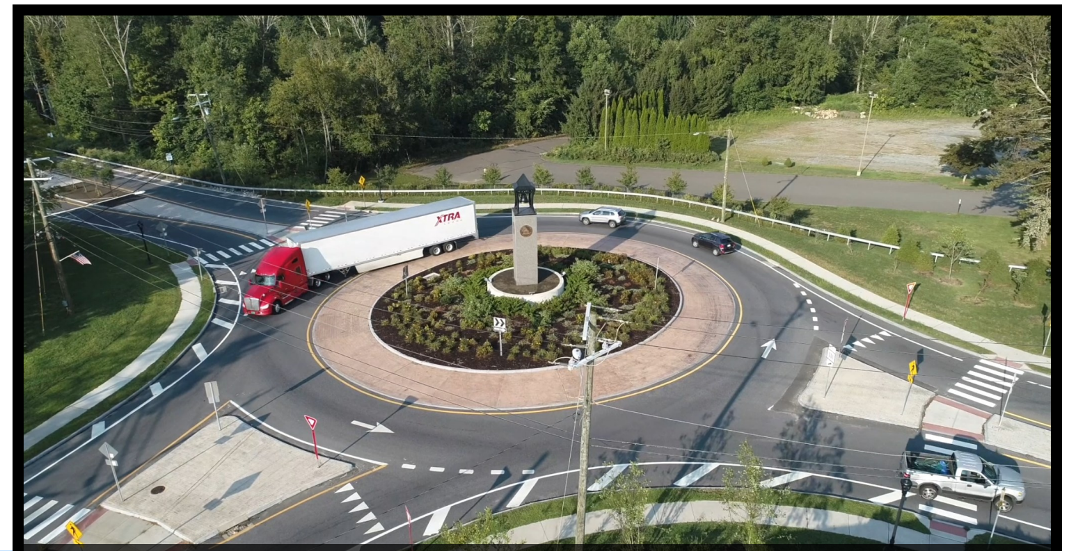
TRUCK APRONS SUPPORT TRACTOR TRAILERS AND FIRE TRUCKS
